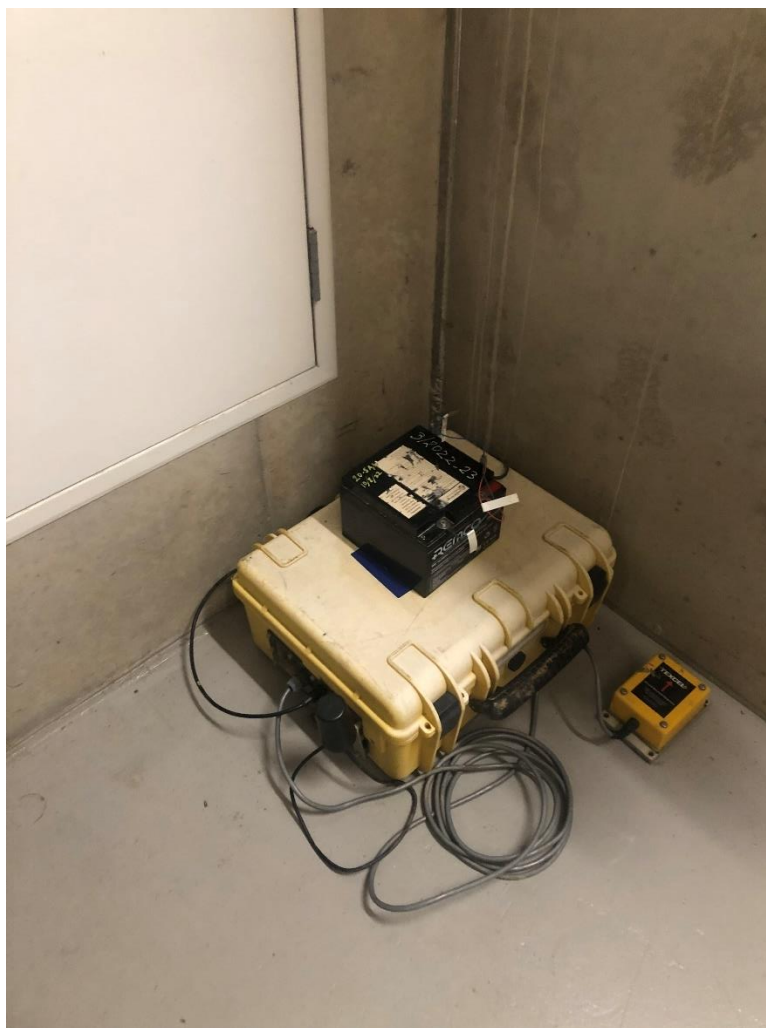
Figure 3 – Location 3 vibration monitor installation (ETM 7418)
