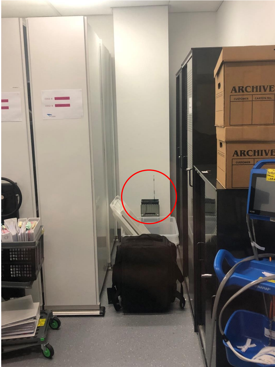
Figure 4 – Location 3 vibration monitor installation (Bruel & Kjaer)
