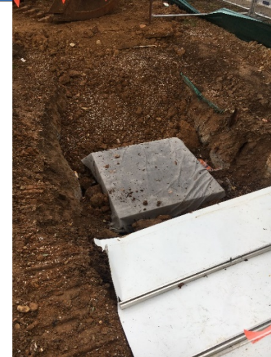
Photo 6 – Erosion and Sedimentation Controls in place
