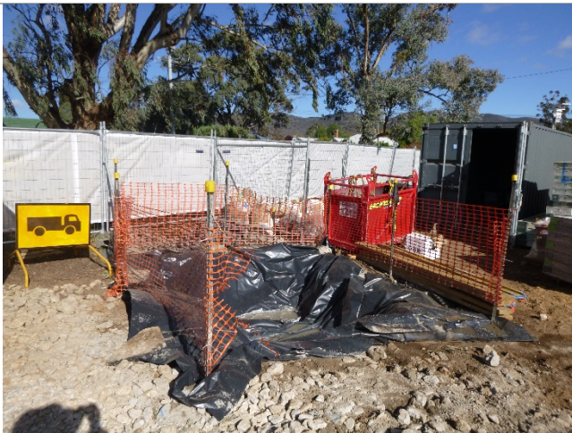
Photo 3 – Concrete washdown area rectified
