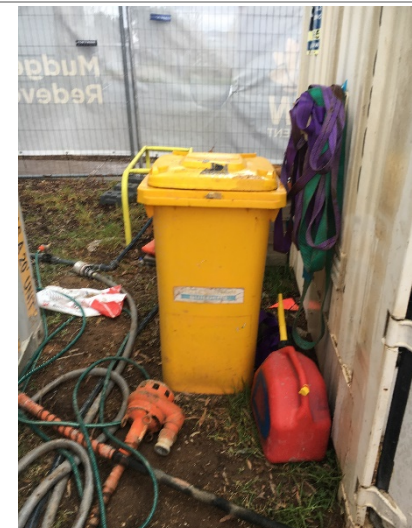
Photo 12 – Spill kit in place next to site office. Other Spill Kit with trip hazards
