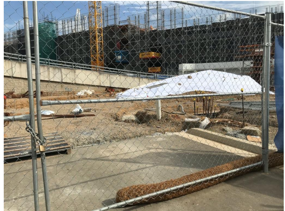
Photo 4 – Other erosion, sediment and dust controls, coir logs in fences and covered stockpile.
