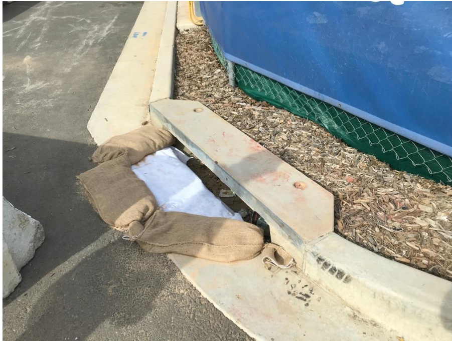
Photo 3 – Erosion and sediment controls around drain pits.
