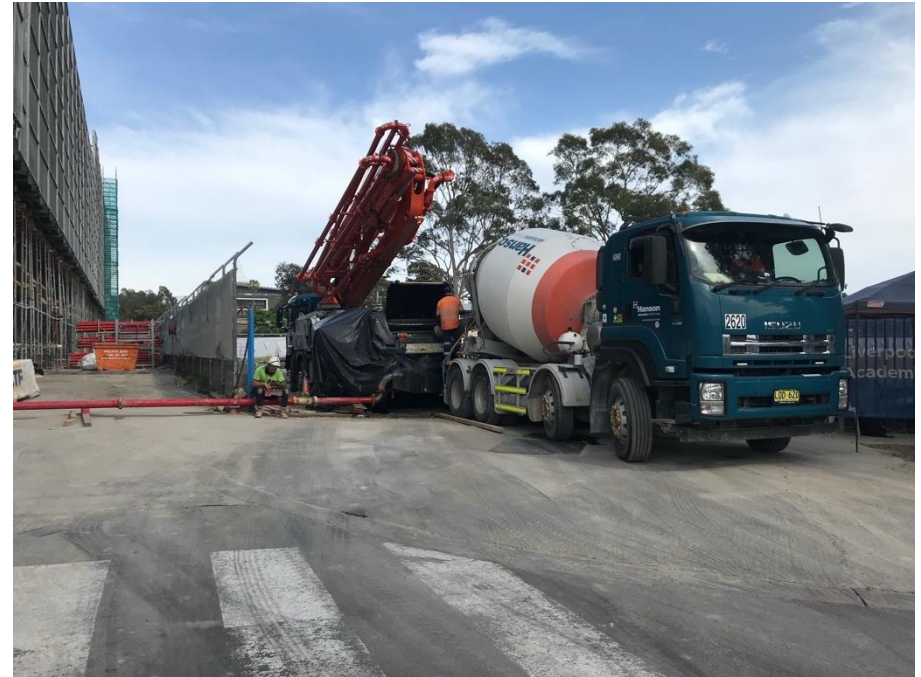
Photo 6 – 'Pumper dump' bin in place to collect excess concrete for off-site disposal.
