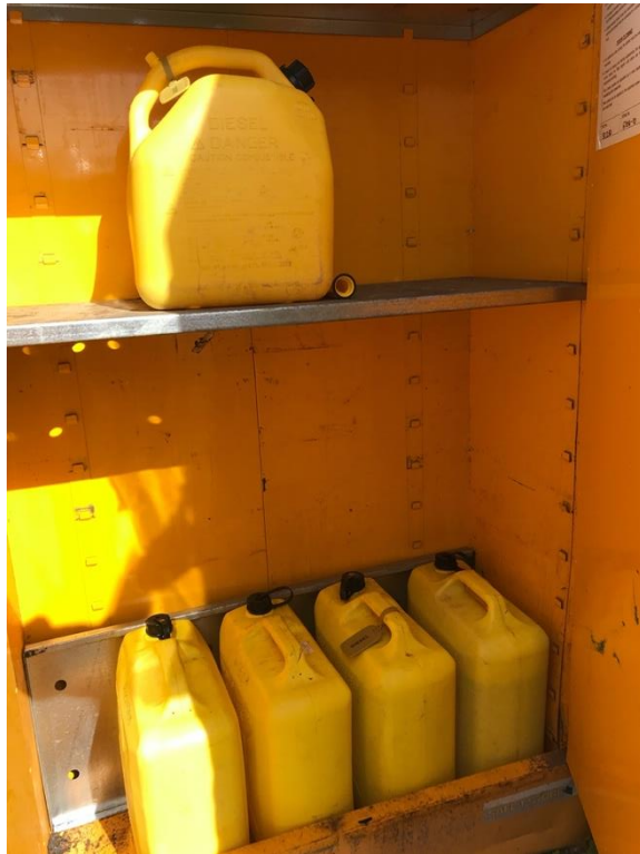
Photo 10 – Secured cabinet for storage of fuel.
