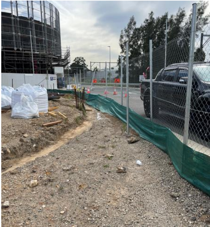
Photo 5 – Silt fence installed around the perimeter of the site.
