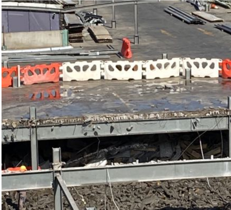
Photo 5 – Demarcation of safety exclusion zone.
