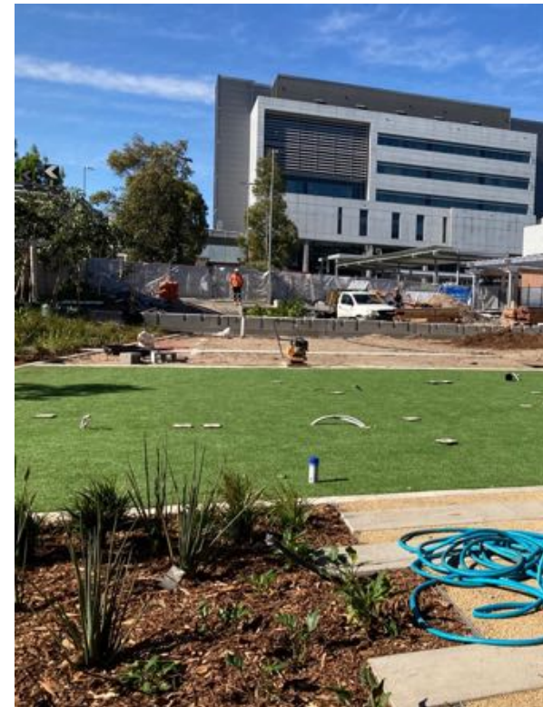
Photo 10 –Landscaping works in progress.
