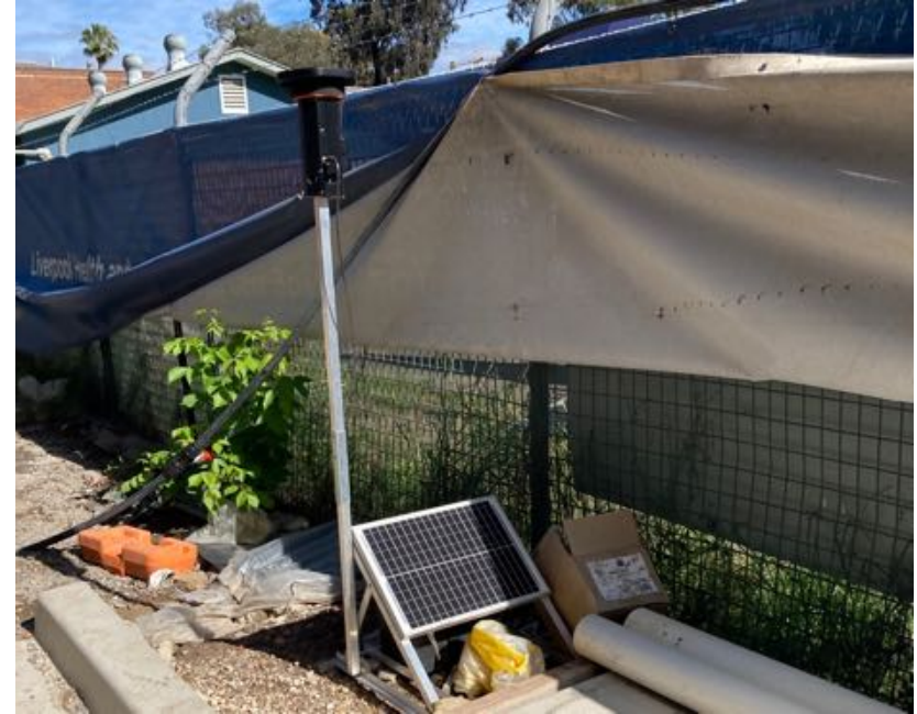
Photo 6 – Noise monitor installed near the demolition area.
