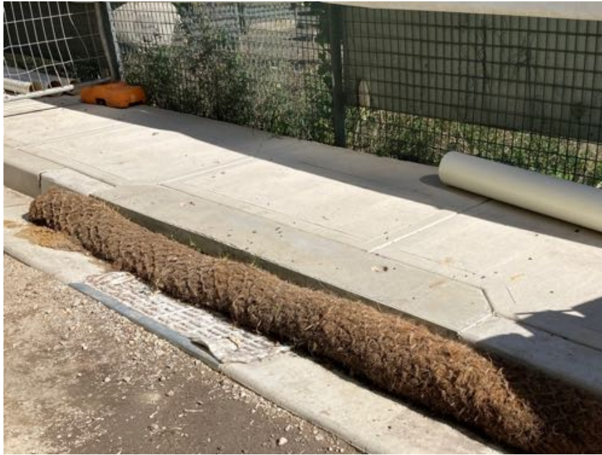
Photo 7 – Drain pits covered for erosion and sediment protection.
