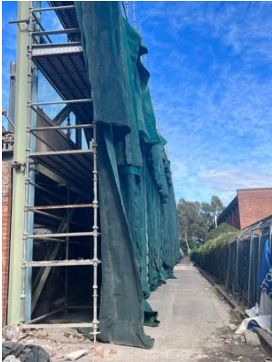
Photo 3 – Green mesh along demolition area for dust protection.
