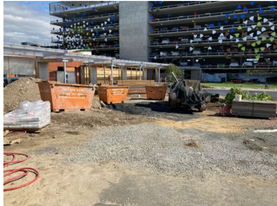
Photo 8 – Waste bins in place around construction areas.
