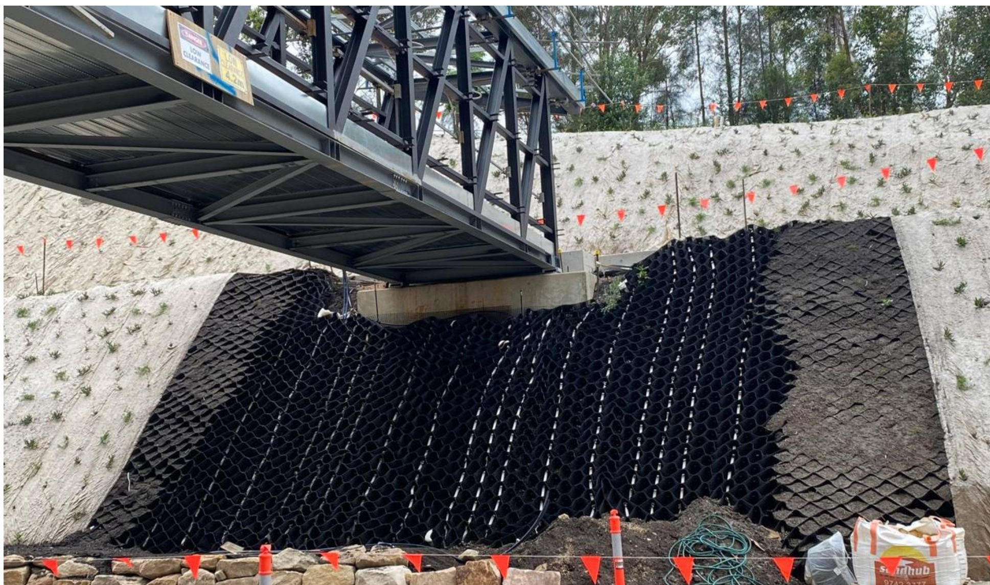
Photo 9: Progressive vegetation and batter stabilisation
