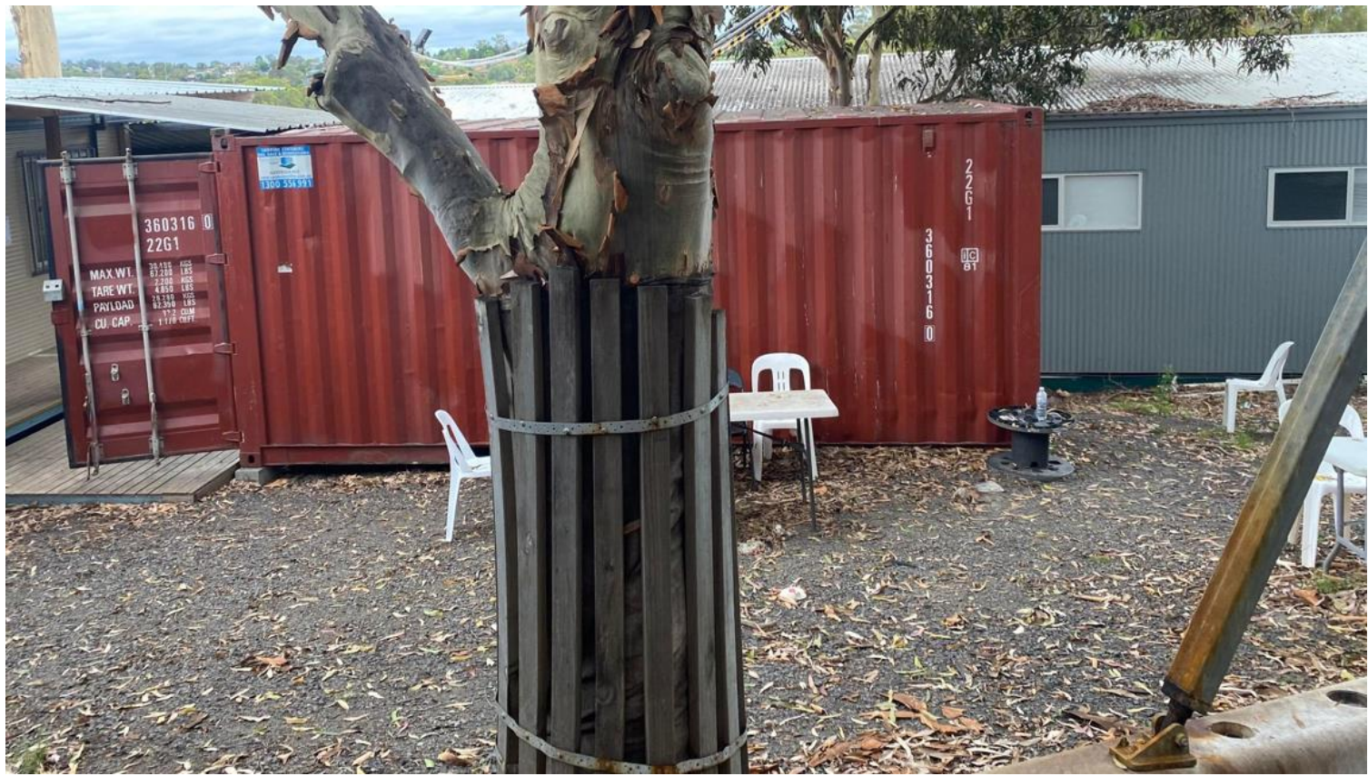
Photo 16: CoC C21 – Temporary tree protection
