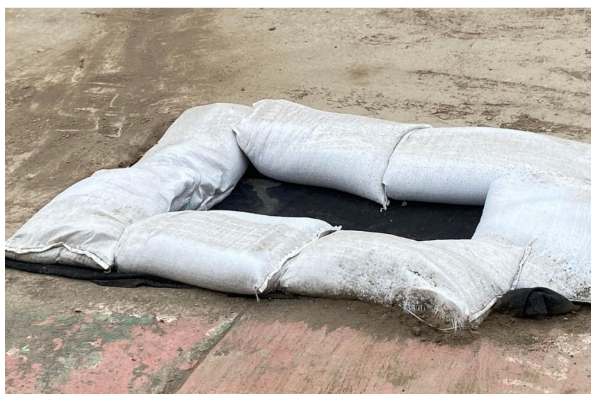
Photo 2 / 2.1: CoC C25 – Sediment control / pit protection
