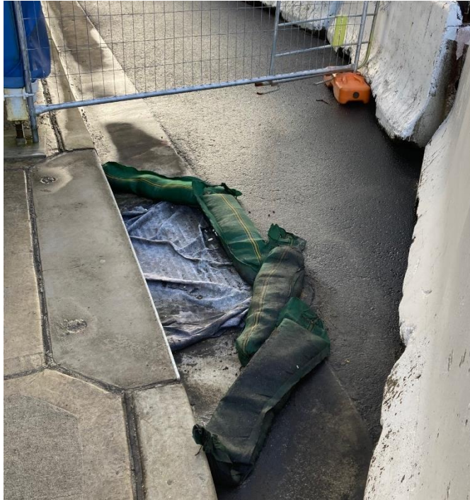
Photo 3 – Erosion and sediment controls around drain pits.
