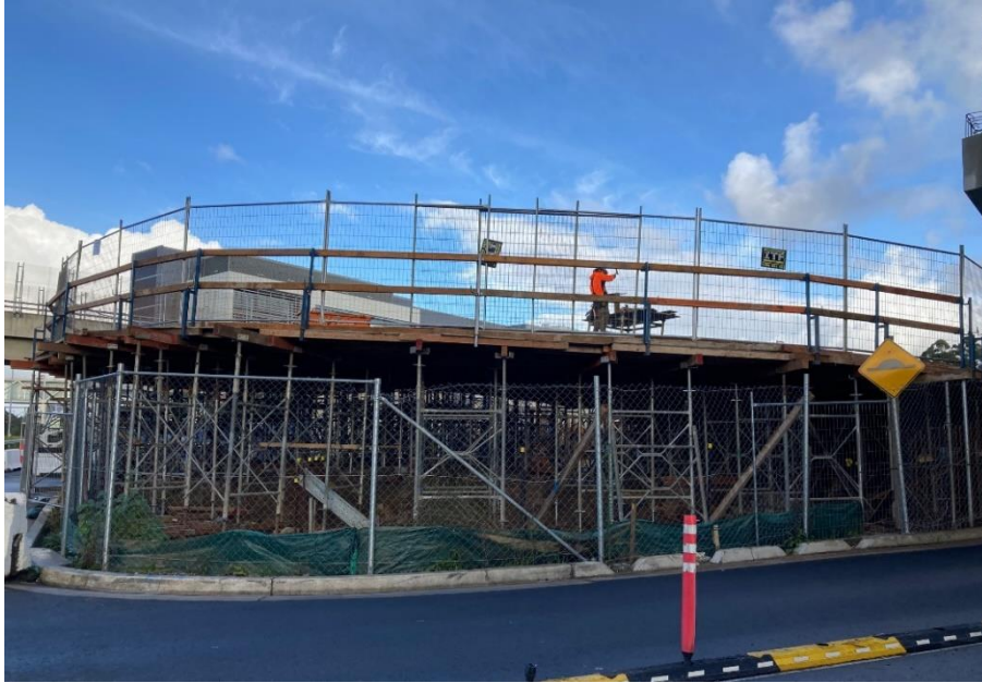
Photo 7 – Structure for car park access ramp. Silt fence installed as erosion and sediment control.
