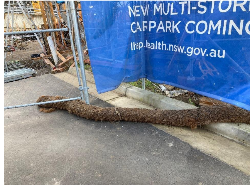
Photo 4 – Other erosion, sediment and dust controls, coir logs placed under gates when not in use.
