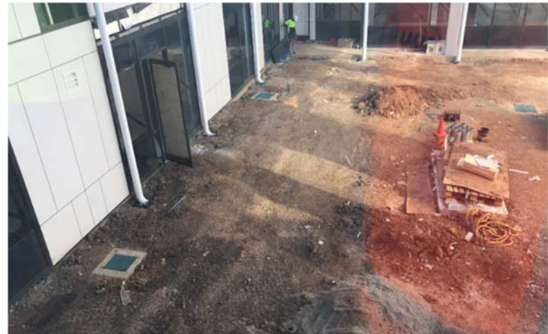
Photo 6 – Pits were covered with mesh screen
