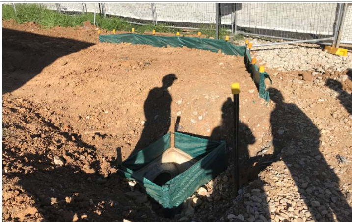
Photo 3 – Sedimentation fence in place at lowest point of the site
