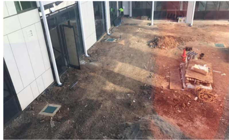
Photo 6 – Pits were covered with mesh screen
