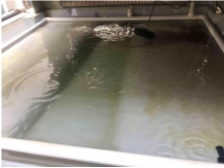
Basin cleaned and over flow cap missing, you can see in picture
