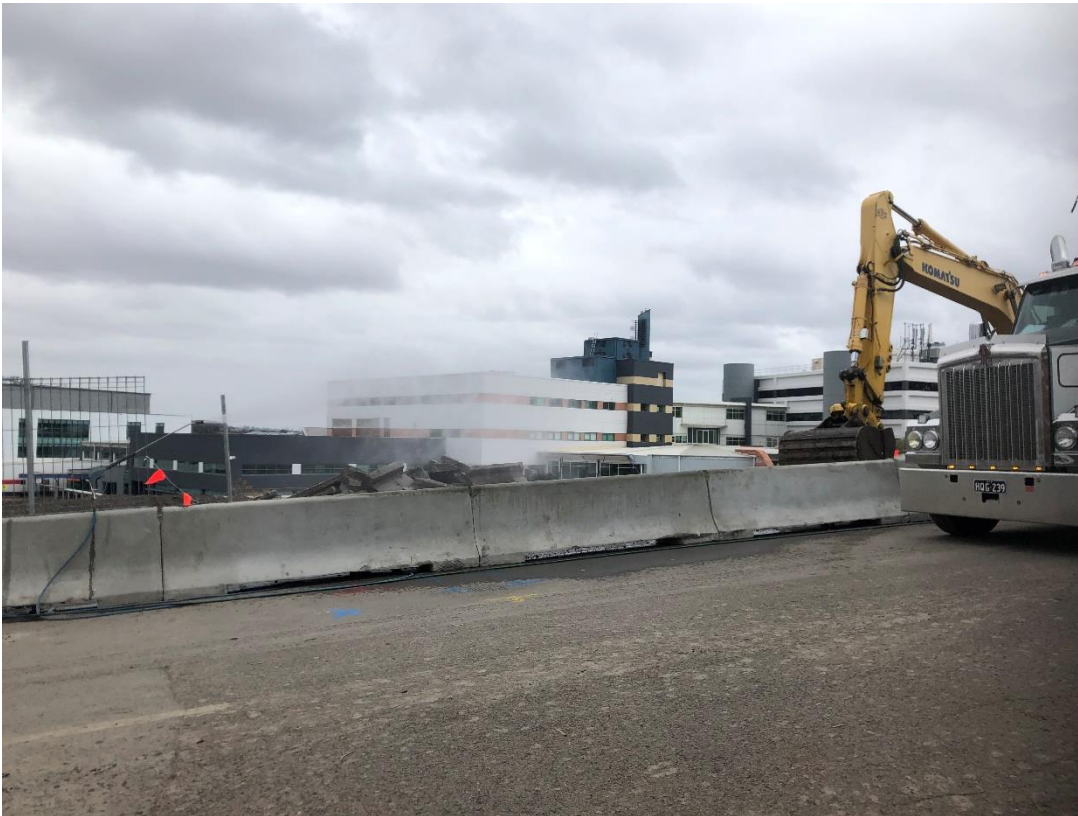
Figure 1: excavation works showing water spray for dust suppression
