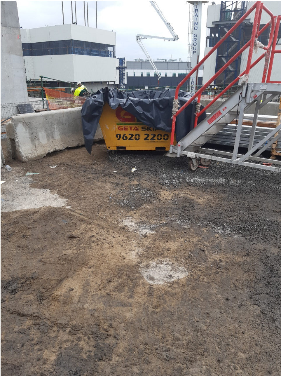
Figure 6: Skips used to store concrete waste prior to removal
