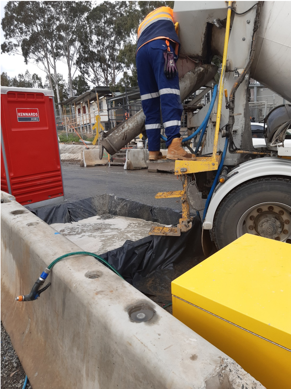
Figure 7: Lined concrete washout
