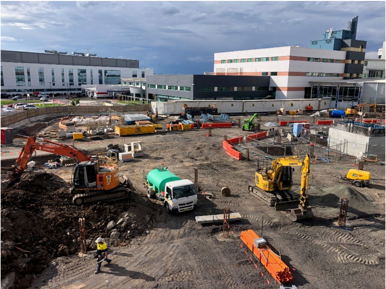
Figure 3: Evidence of water cart in site in early concreting works.
