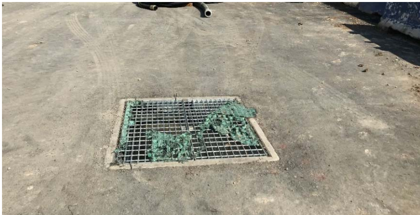
Photo 7 – Sediment cover of the pit needs to be replaced.
