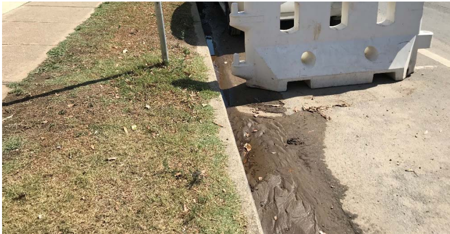
Photo 5 – Accumulated silts along the gutter to be removed.
