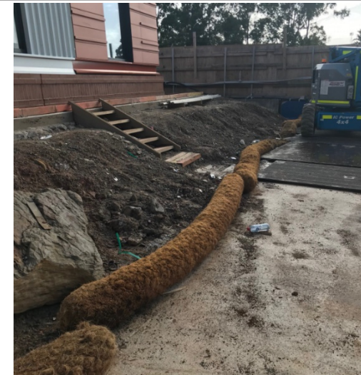
Photo 8 – Sediment controls in place.
