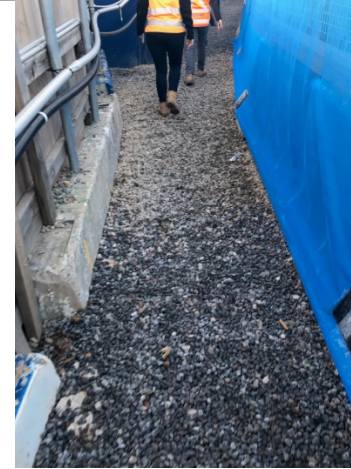
Photo 2 – Entrance corridor with rock lining controls.
