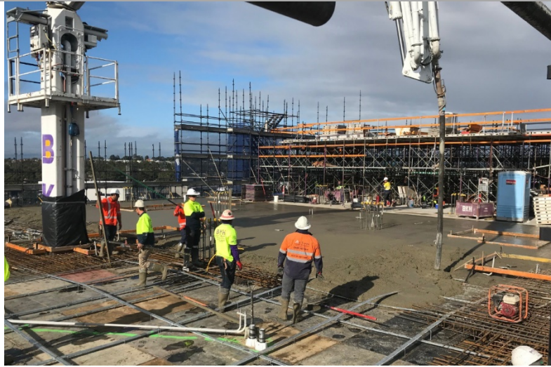
Photo 5 – Concrete pouring works.
