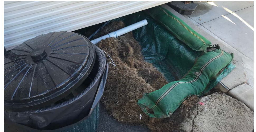
Photo 12 – Sediment controls were installed around stormwater pits.
