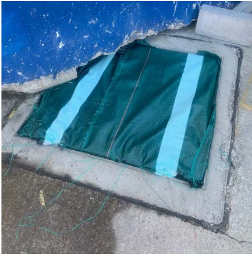
Photo 9 – Drain with geo-fabric at the entrance of North Road
