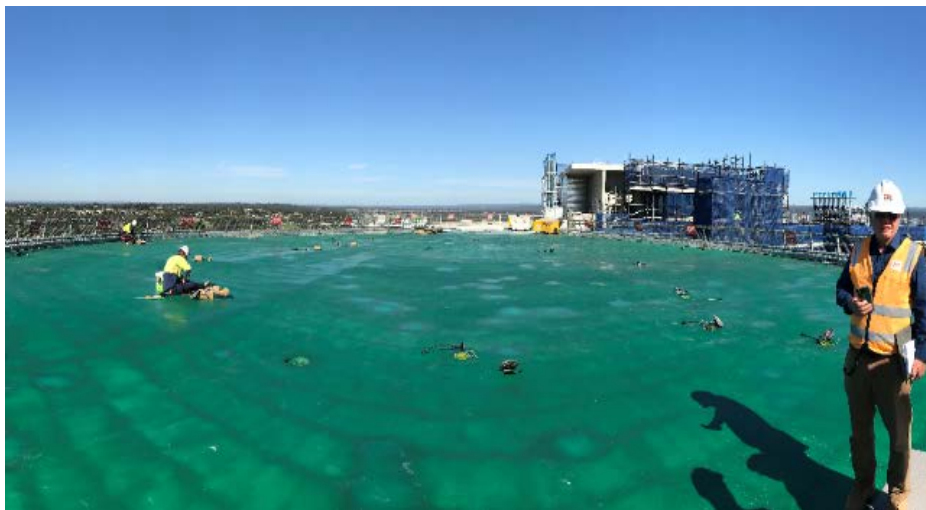
Photo 15 – Installation of lights at the Helipad
