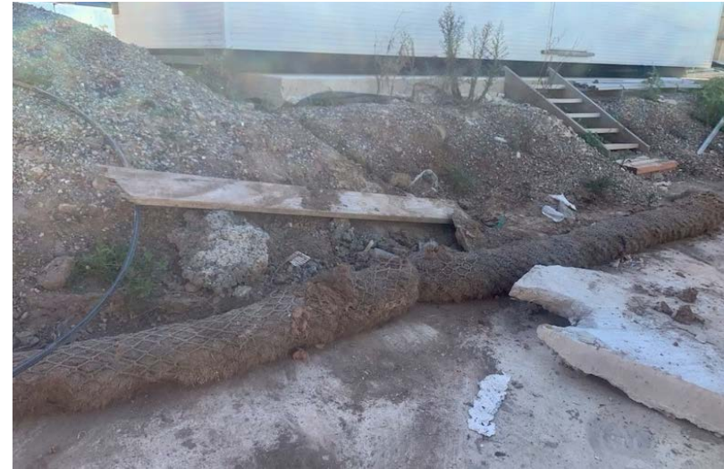
Photo 10 – Adjustment of silt socks at the western end of North Road
