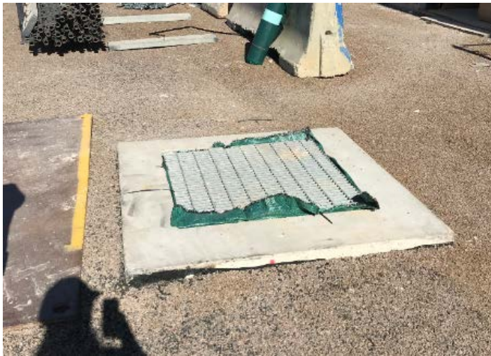
Photo 5 – Sediment controls in place around stormwater pits
