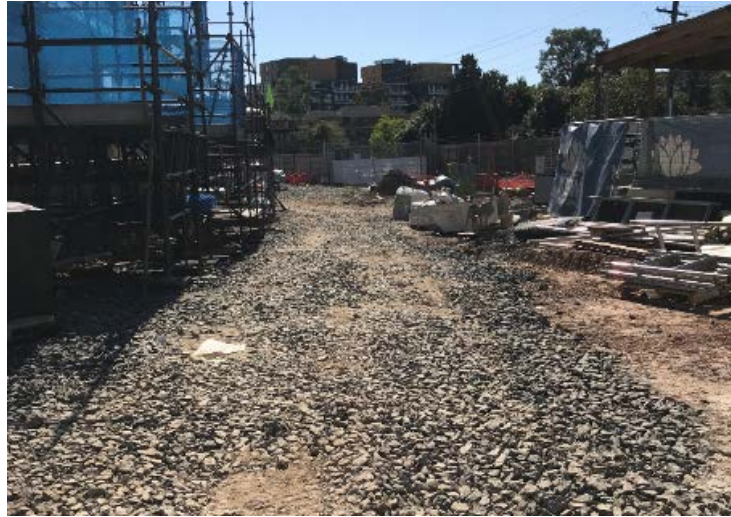
Photo 1 – Ambulance bay with rock lining controls
