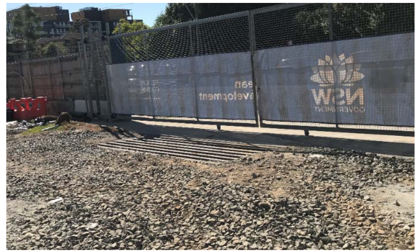
Photo 14 – Rumble grid was in place at the site entrance
