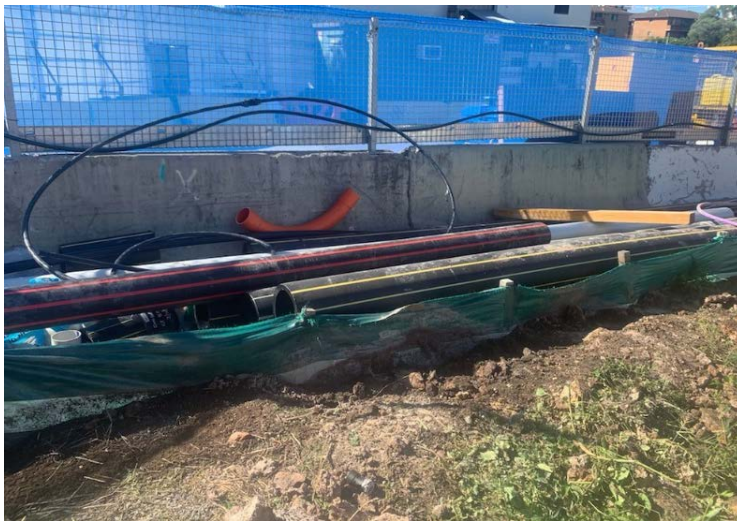
Photo 11 – Slit fence rectified in the ambulance bay area
