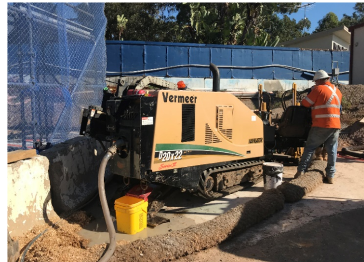
Photo 8 – Directional drilling works with sediment controls
