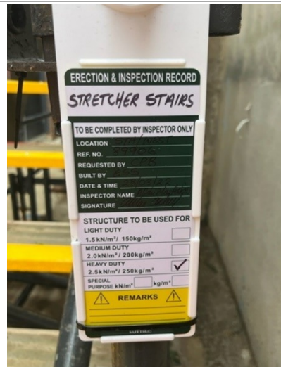
Photo 11 – Scaffold tagged and steps with anti-slip
