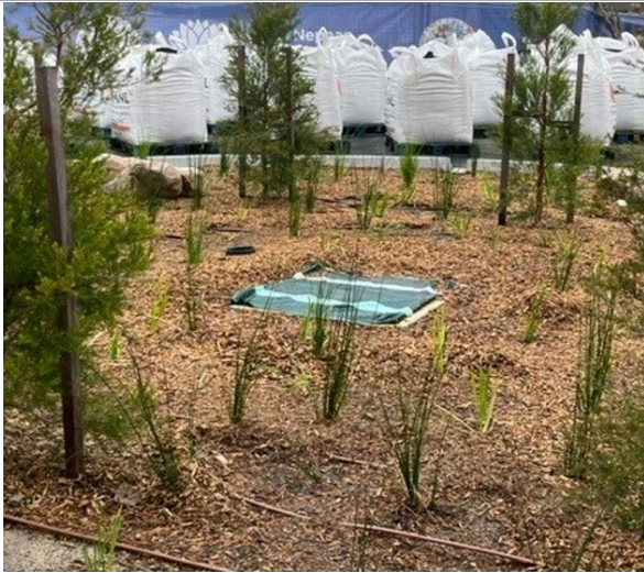
Photo 5 – Drain with geo-fabric at the landscaping works area
