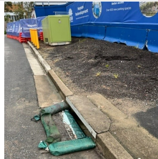
Photo 6 – Stormwater pit with geo-fabric and sandbags
