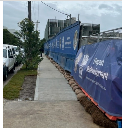
Photo 2 –Erosion and sediment controls (sandbags) along the site boundary
