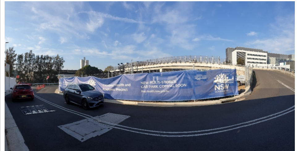
Photo 2 – Road kept clean free from dust and mud.
