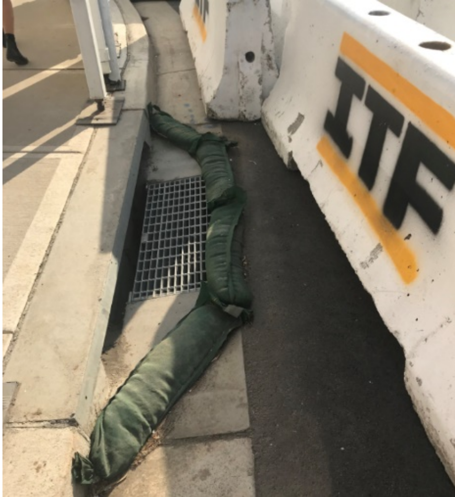
Photo 5 – Outside pits protected with sandbags.
