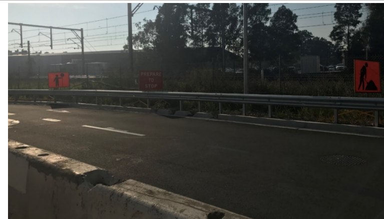
Photo 4 –Traffic controls in place.
