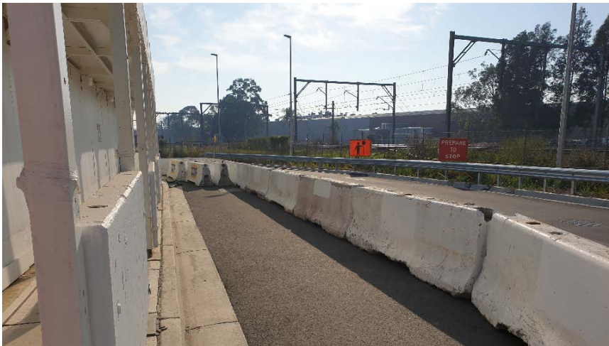
Photo 9– Jersey barriers were installed to separate pedestrian from construction traffic.
