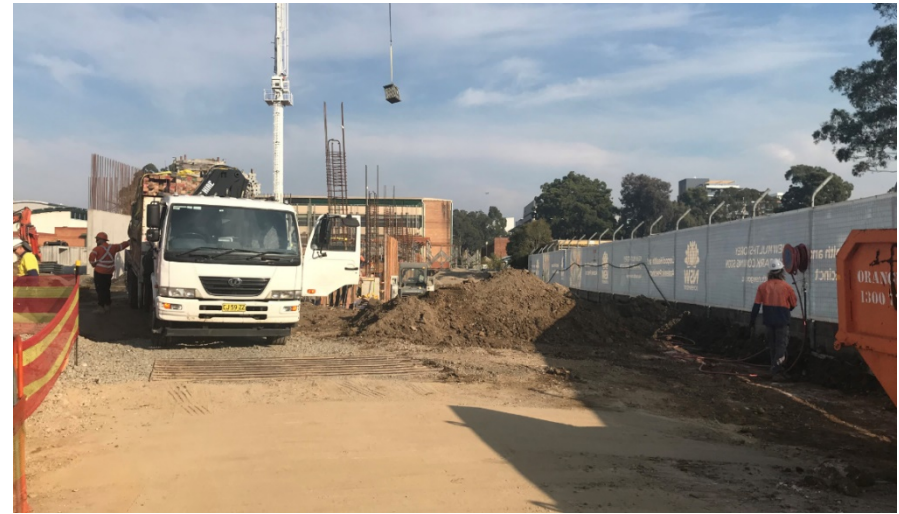
Photo 8 – Rumble grid was installed at the site entrance/exit.
