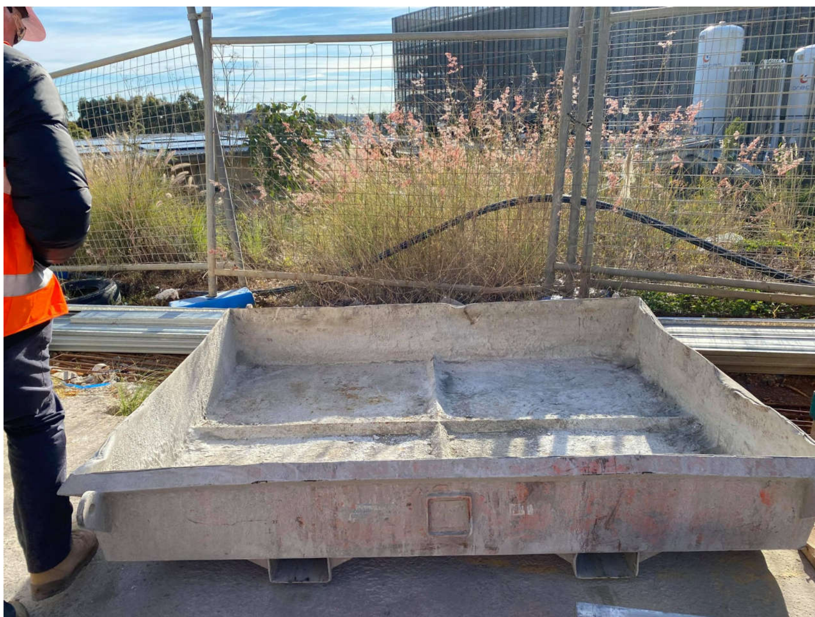
Photo 8: CoC C33 – Concrete washout trays
