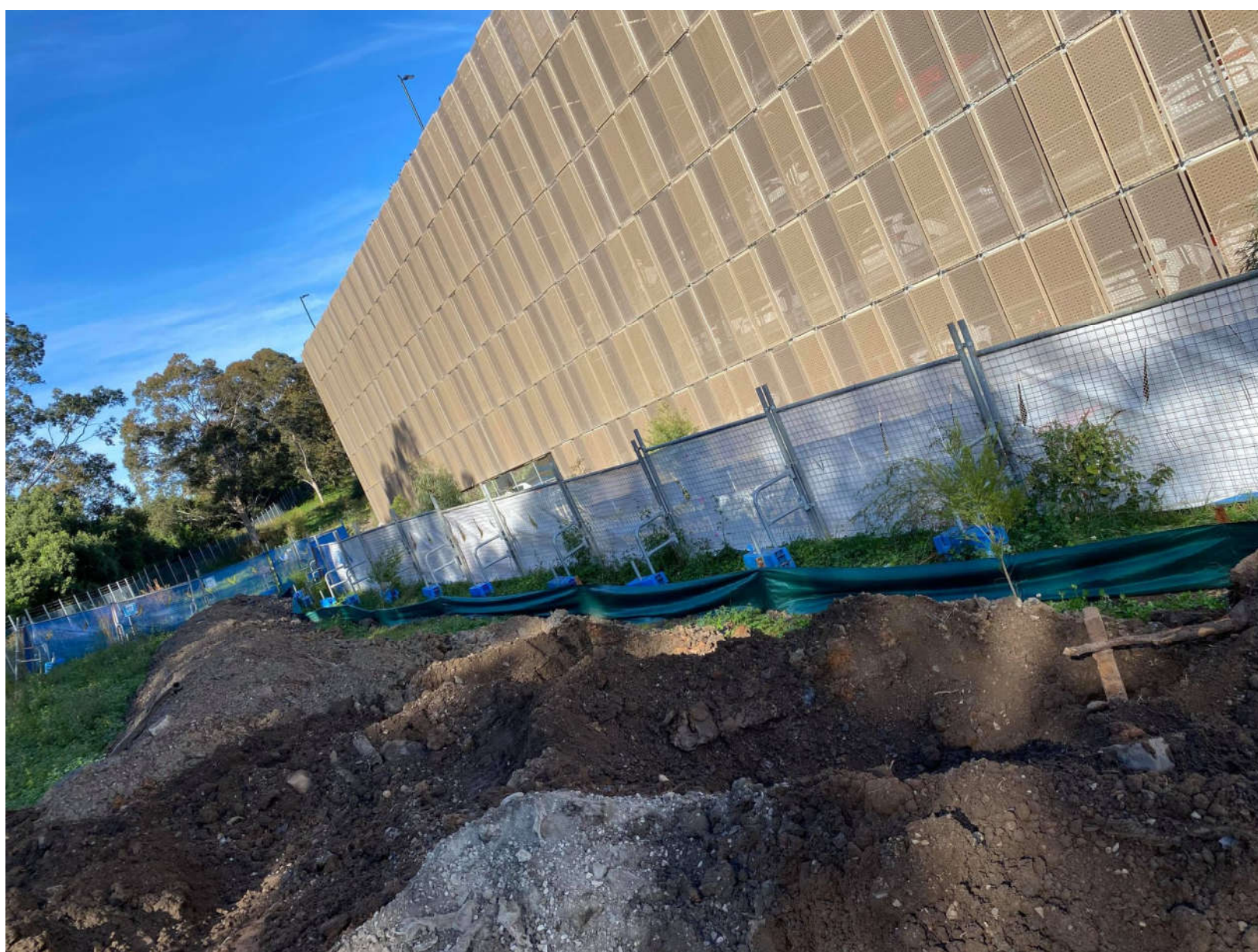
Photo 6: CoC C25 – Erosion and sediment control
