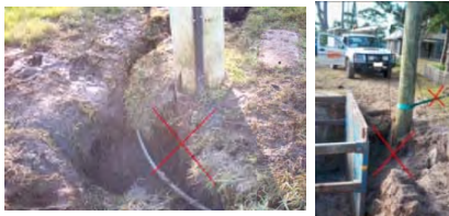
Above: Poles with become unstable if undermined
