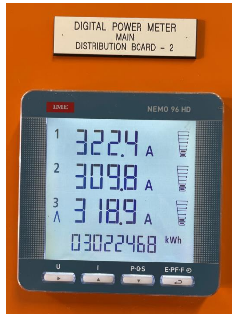
Figure 4-3: Maximum Demand Reading of the Incoming Supply of MDB2
