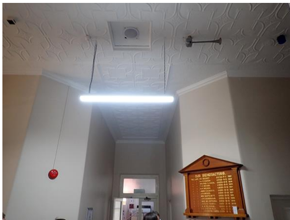
5 Interior view west through the main hallway.
