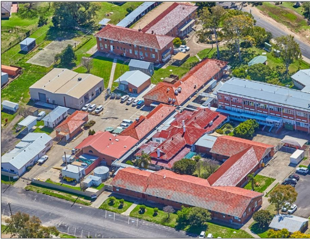
Aerial view of Moree Hospital.
