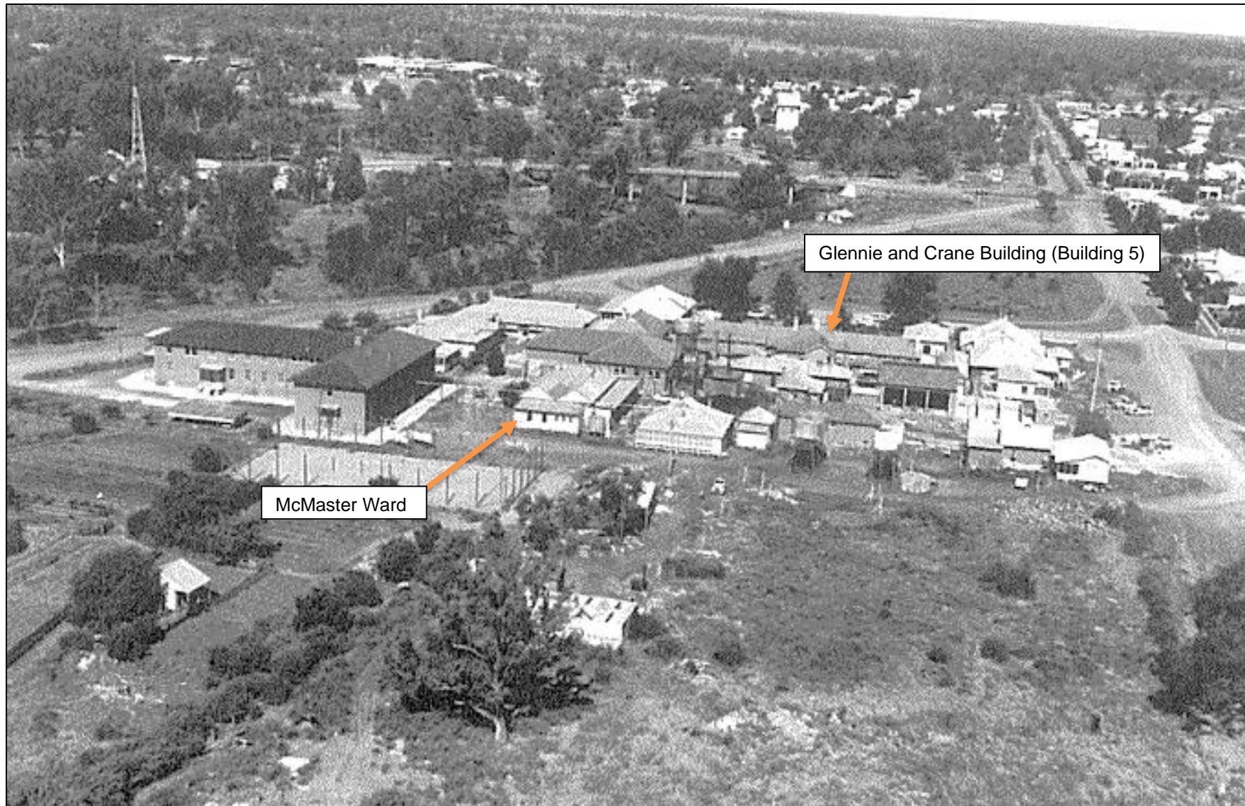
Figure 2-4: Aerial image showing the Moree Hospital from the west after 1971 (Source: Briggs Smith 2003).
