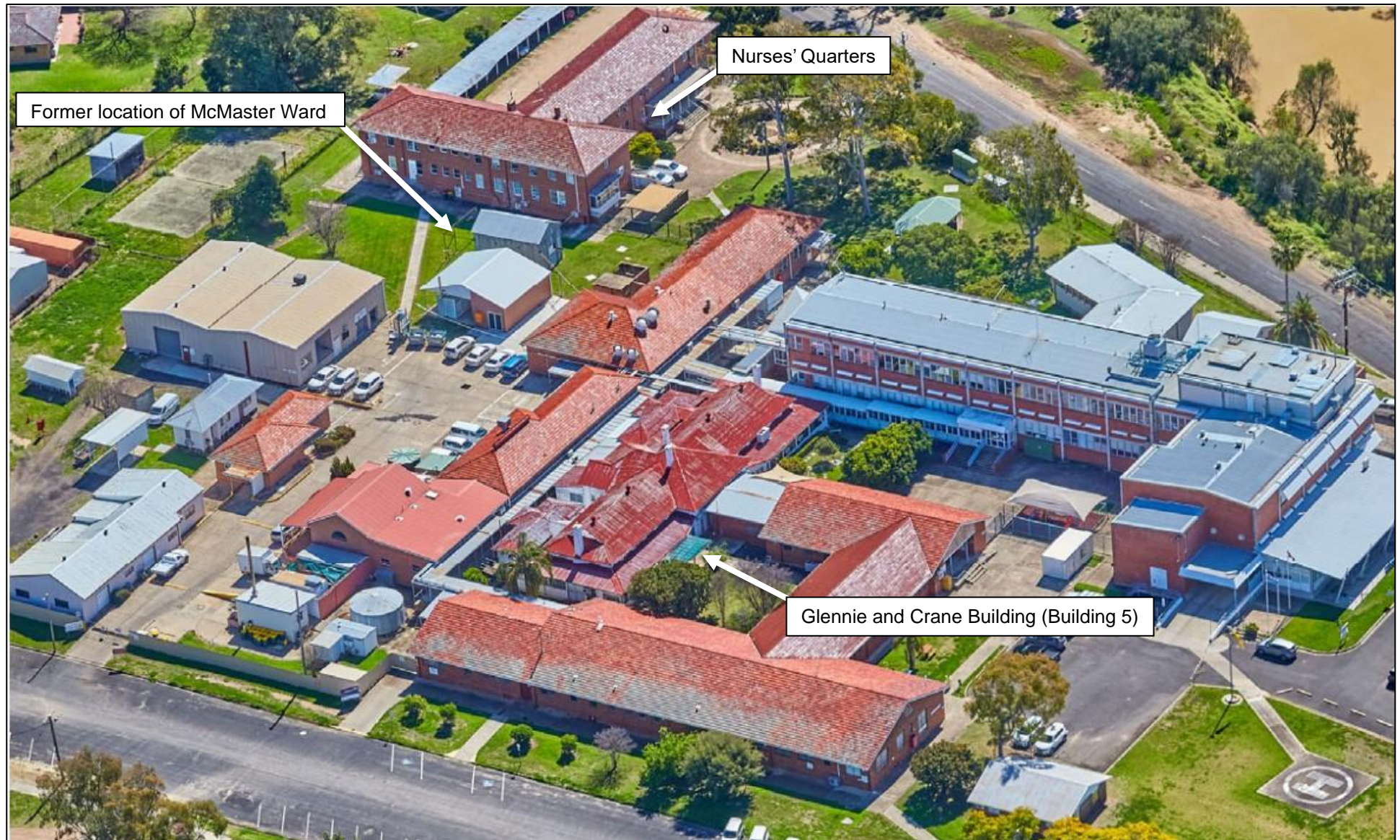
Figure 2-3: Aerial image from the southwest showing the Moree Hospital and key items (Source: NSW Health Infrastructure).
