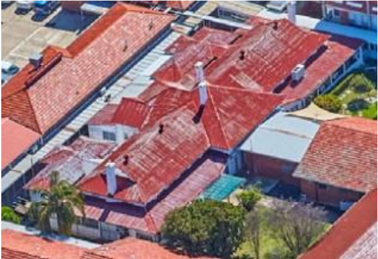
Figure 3-2: Views of the Glennie and Crane Building during the assessment.
