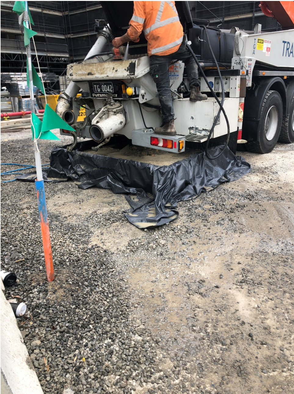
Figure 5: Lined concrete washout
