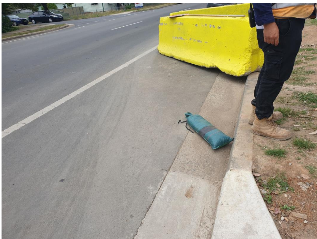
Photo 4: Somerset Street sediment control.
