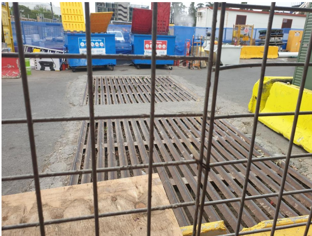
Photo 5: Site access rumble grids.
