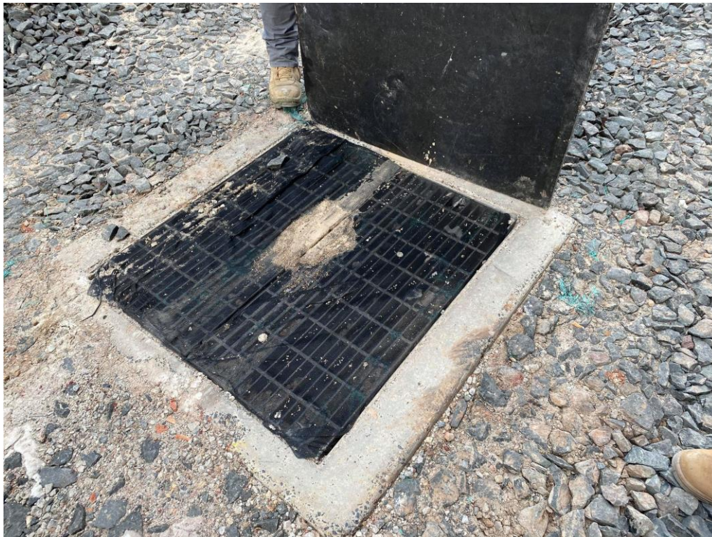
Photo 6: Stormwater pits protected from sediment runoff with a steel plate and silt cloth underneath.
