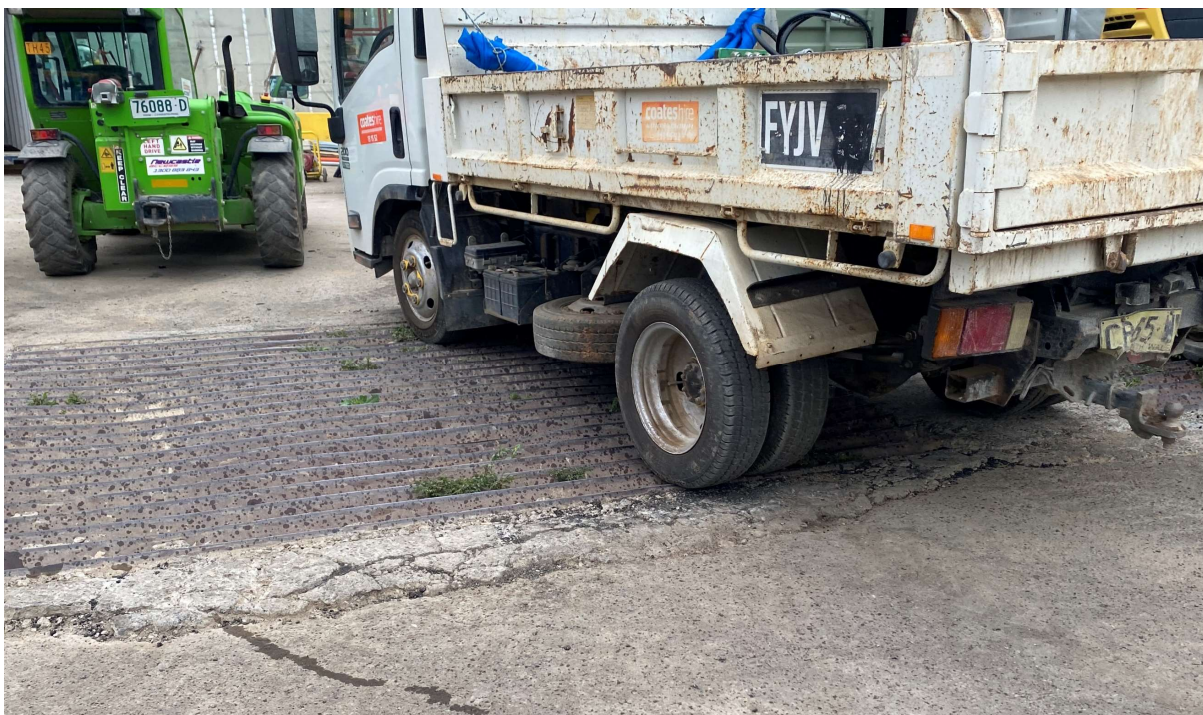
Figure 9: Rumble grid at site entrance on Somerset Street
