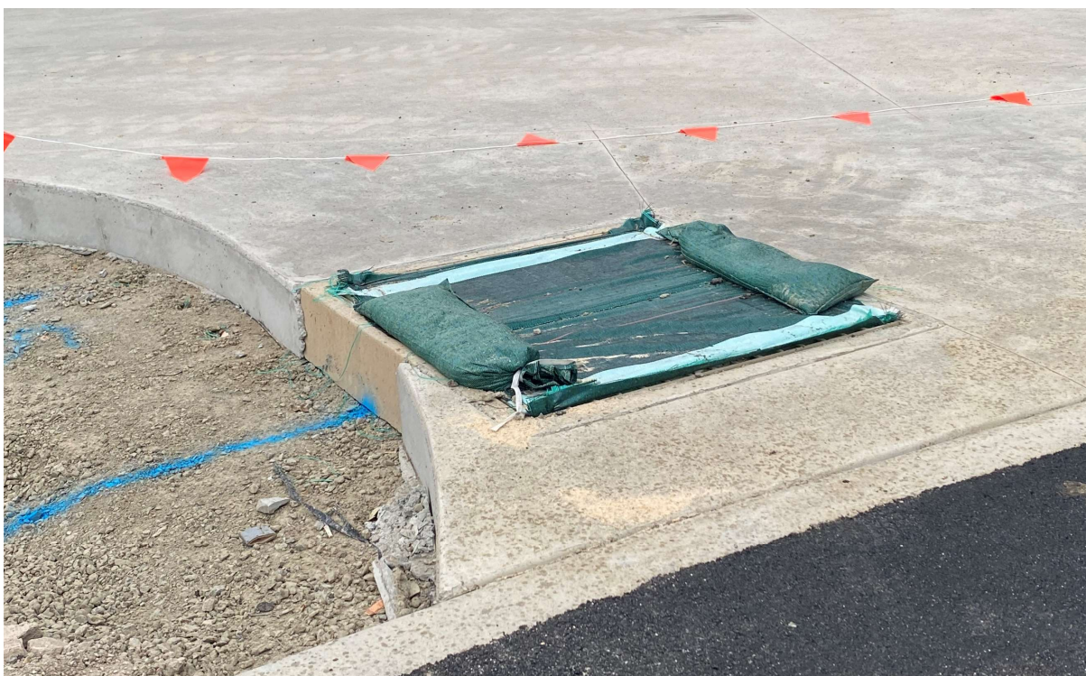
Figure 10: Example of sediment controls protecting active stormwater drains onsite
