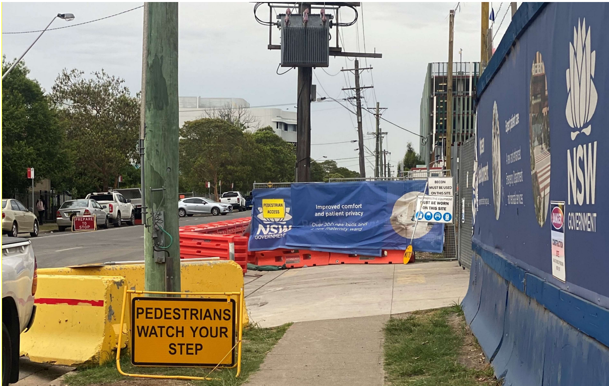
Figure 3: Site hoarding and pedestrian access arrangements
