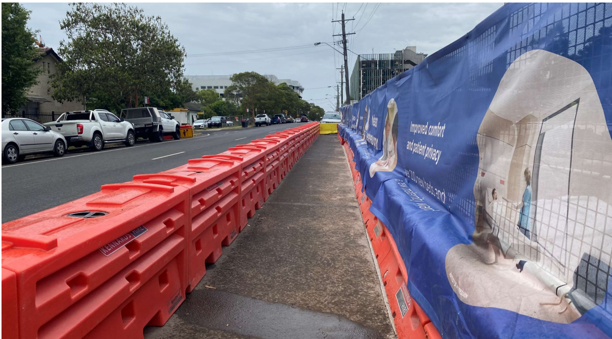
Figure 4: Temporary fencing along site perimeter on Somerset Street with NSW Health shade cloth, and pedestrian access delineation
