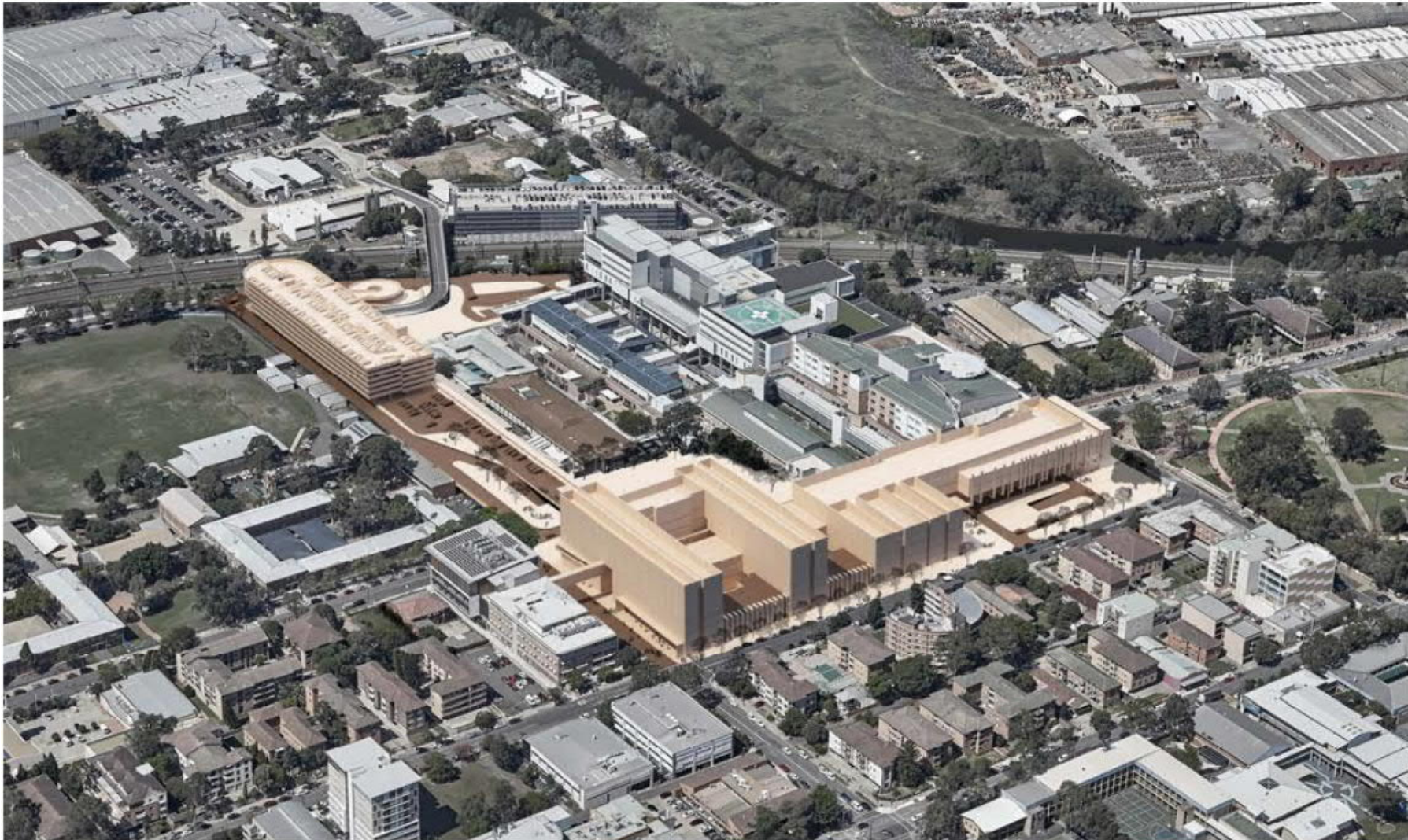
Figure 2: Liverpool Hospital Redevelopment artists redevelopment, viewed from the north-west of the site
