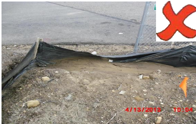
Sediment fence requires maintenance
