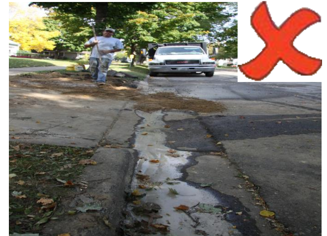
Cement wash-off flowing to kerb
