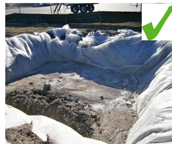
A simple but effective plastic and geofabric-lined washout area.
