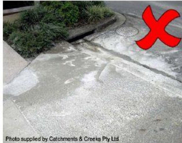
Cement wash-off from concreting works
