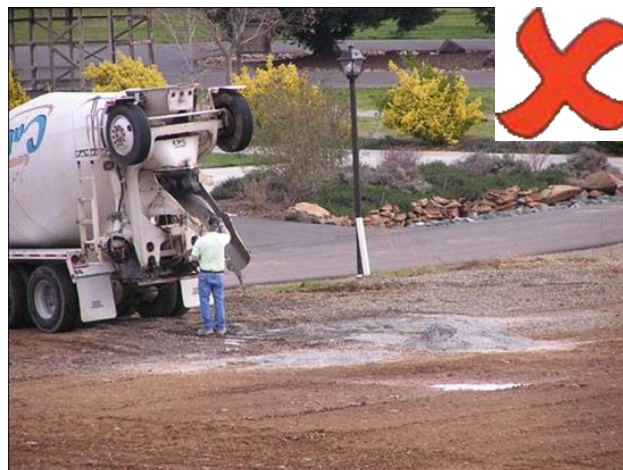
Concrete washout directly onto the ground. This substance can leach / run-off to contaminate soils and water bodies.
