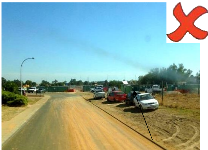
Dirt has been tracked extensively onto a public road. This can become airborne or enter stormwater drains.
