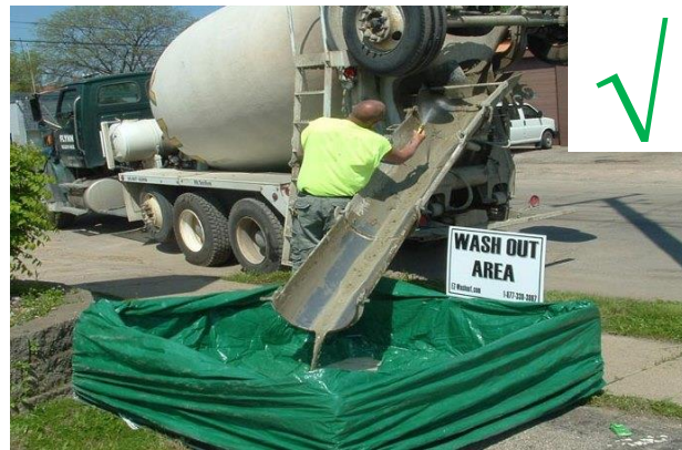
Sufficient Concrete wash bay
