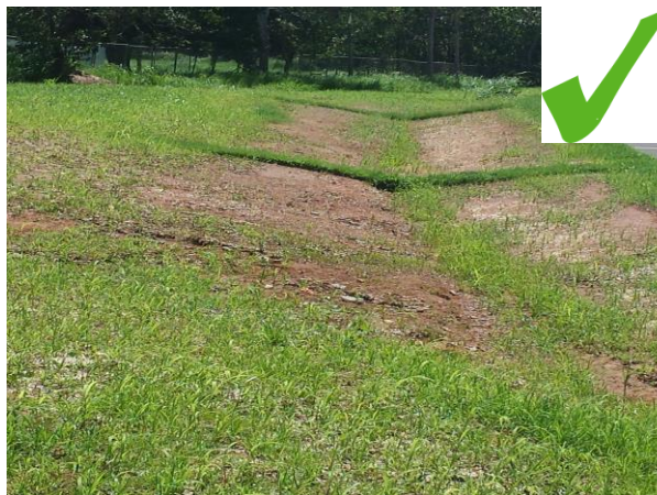
Revegetation of previously exposed swale drain. A mixture of hydromulch and turf has been used.
