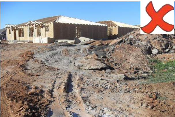
Insufficient concrete wash bay Concrete residue is not retained within bunded area
