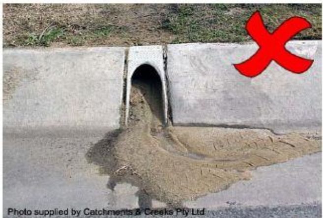
Sediment released from stormwater pipe
