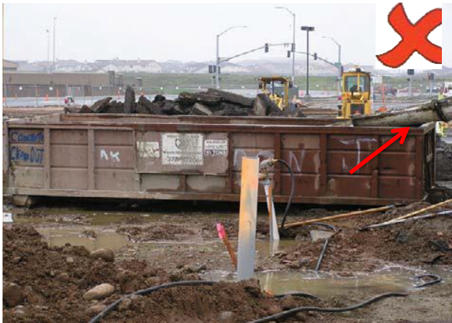
The red arrow points to a ready mixed truck chute that's being washed out into a roll-off bin, which isn't watertight. Leaking wash water, shown in the foreground, will likely follow similar paths to nearby surface waters.
