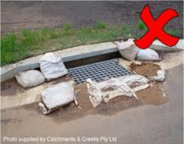
Sand bags need to be replaced
