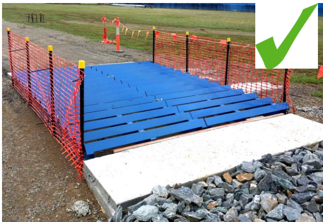
Rumble grid and rock pad in place on the construction site exit.
