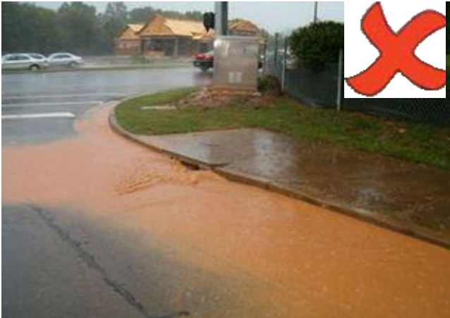
Contaminated stormwater run-off from construction site
