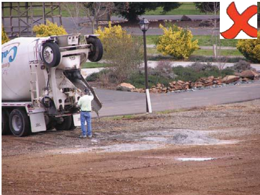
Wash water being dumped on the ground
