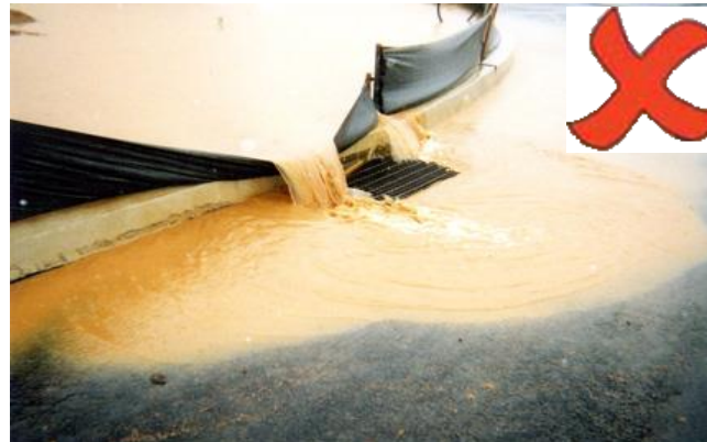
Sediment fence over flow
