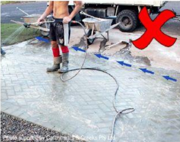
Cement wash flowing to kerb
