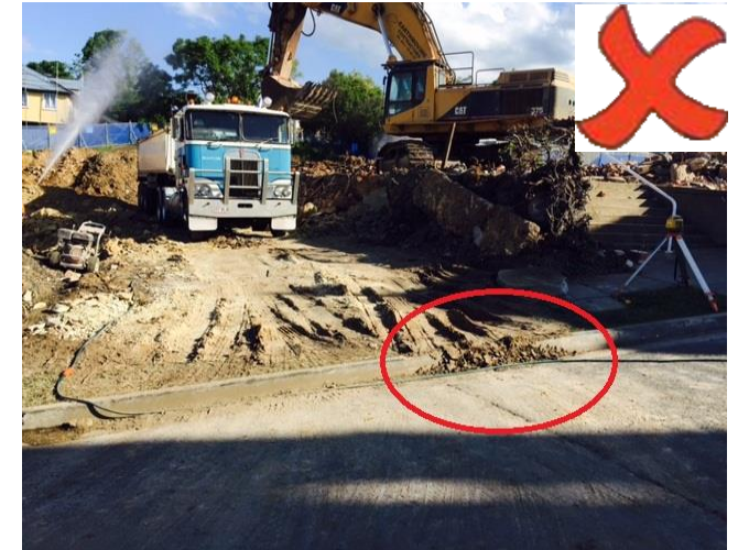
Site entry point not stabilised
