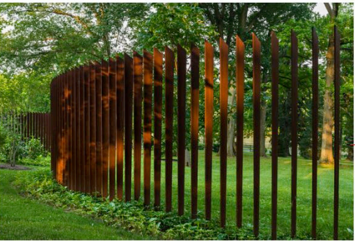
CORTEN STEEL VERTICAL FENCE & SCREEN - GAP BETWEEN TO BE LESS THAN 100mm
