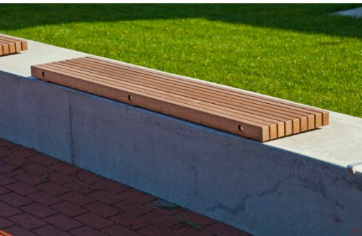
MODWOOD DECKING TO TOP OF MASONRY BLOCK WALLS BEACH SEATS
