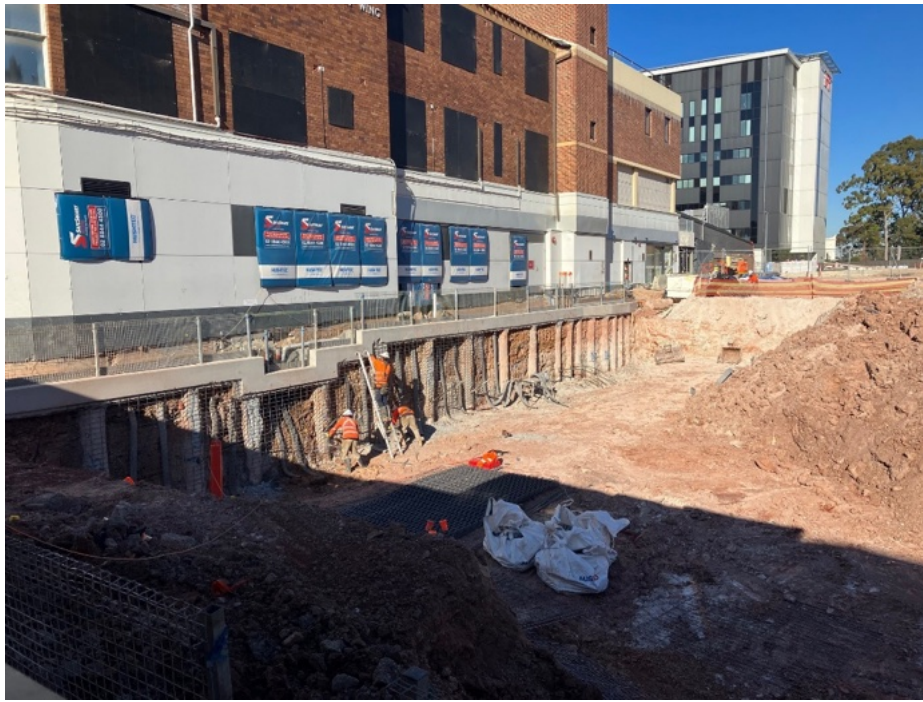
Photo 9 – Noise blankets installed along JH Bart Wing.
