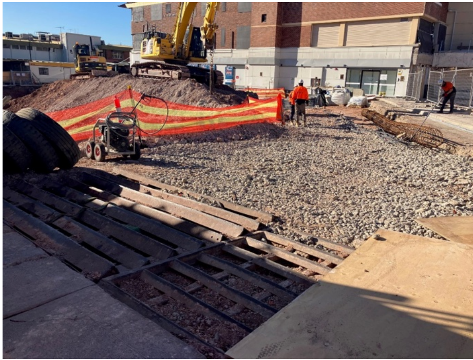
Photo 11 – Rumble grid and high pressure water hose at heavy vehicle access. Rock used for stabilisation.
