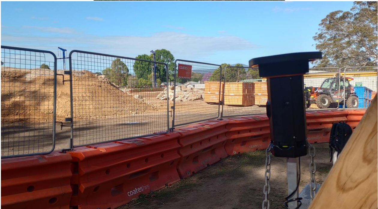
Figure 4 – HEX000401 – Pre-School Boundary Fence Near Outdoor Play Area
