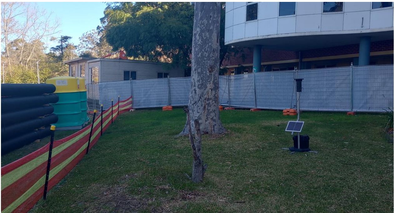
Figure 3 – HEX000232 – West of Early Works Zone Near Block A
