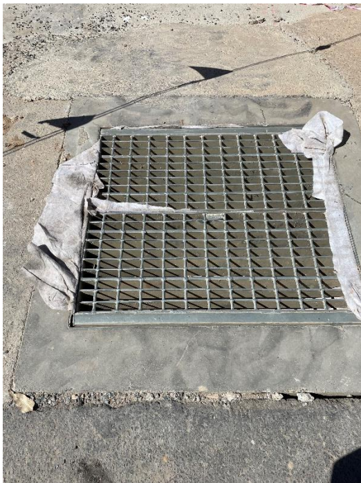
Figure 3: Geofabric lined drainage pits
