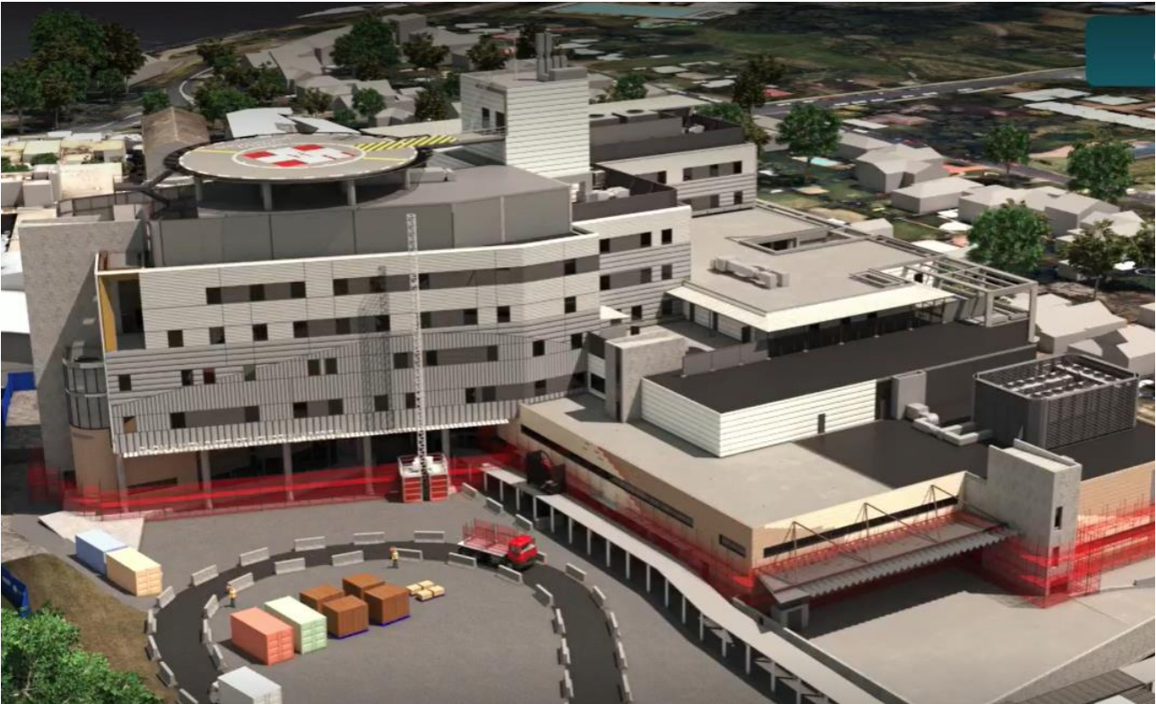
Figure 7 Shoalhaven Hospital Façade and Fitout
