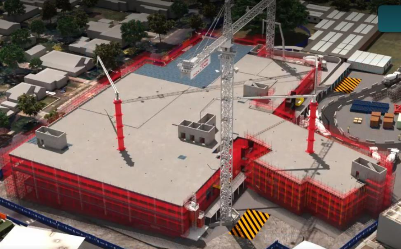
Figure 5 Shoalhaven Hospital Superstructure L1 – L4 Inc. Service Rough In
