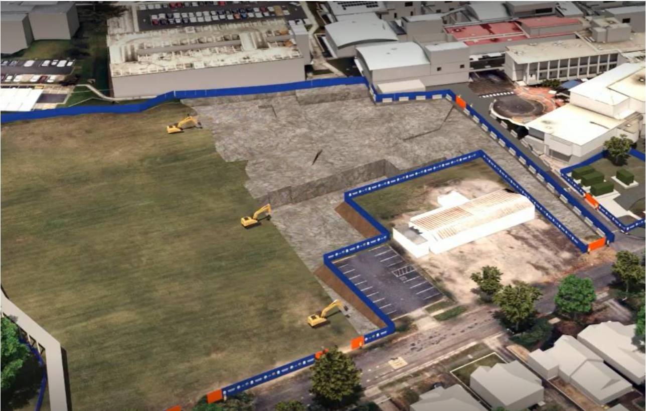
Figure 3 Shoalhaven Hospital Bulk Excavation
