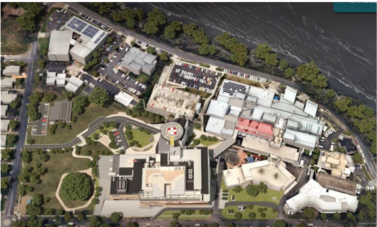
Figure 8 Shoalhaven Hospital Landscaping and External Works
