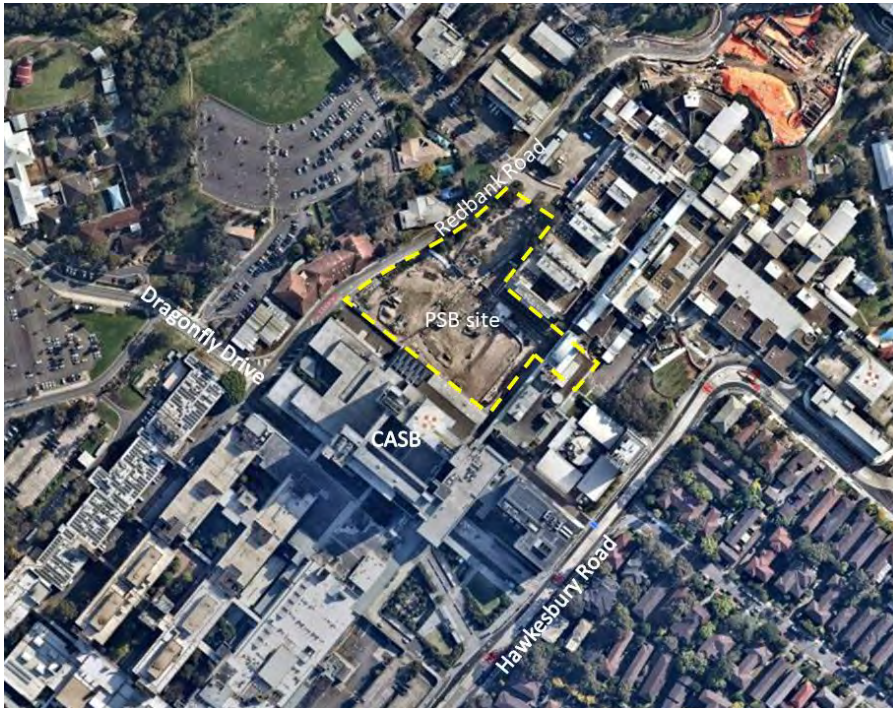
Figure 1 Building aerial showing the PSB development site including site compound
