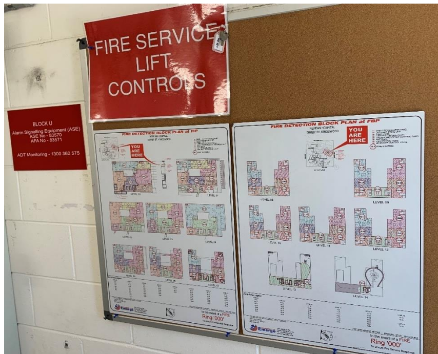
Photo 5 – Fire Detection Block Plans in Fire Control Room
