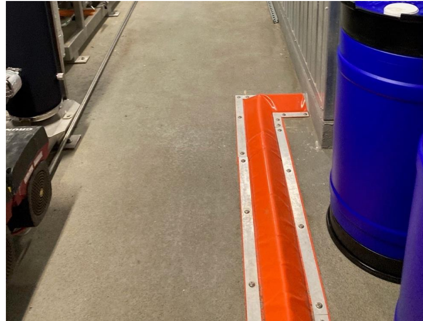
Photo 8 – No drains in the area around stored chemicals
