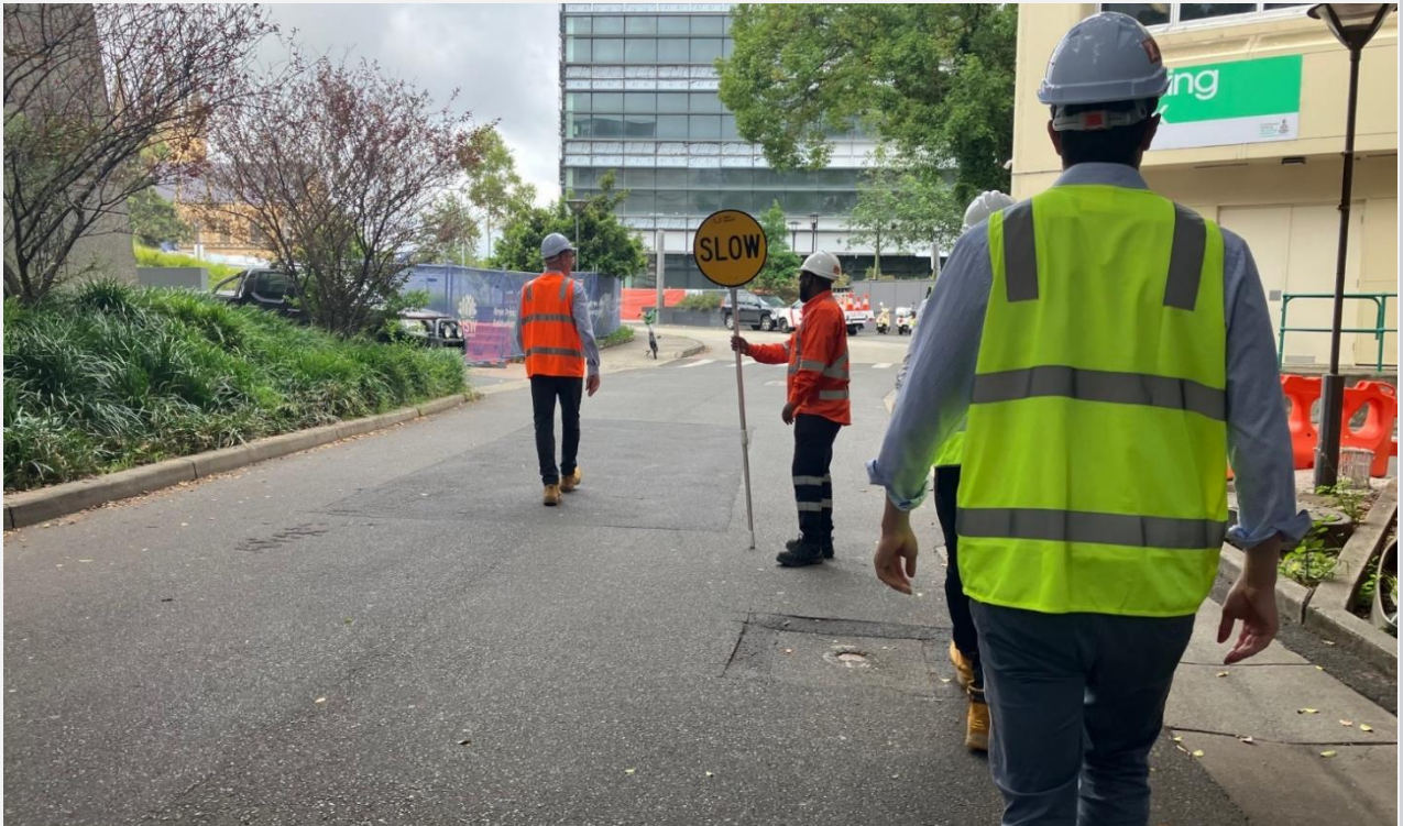
Traffic controller in place at Lambie Dew Drive
