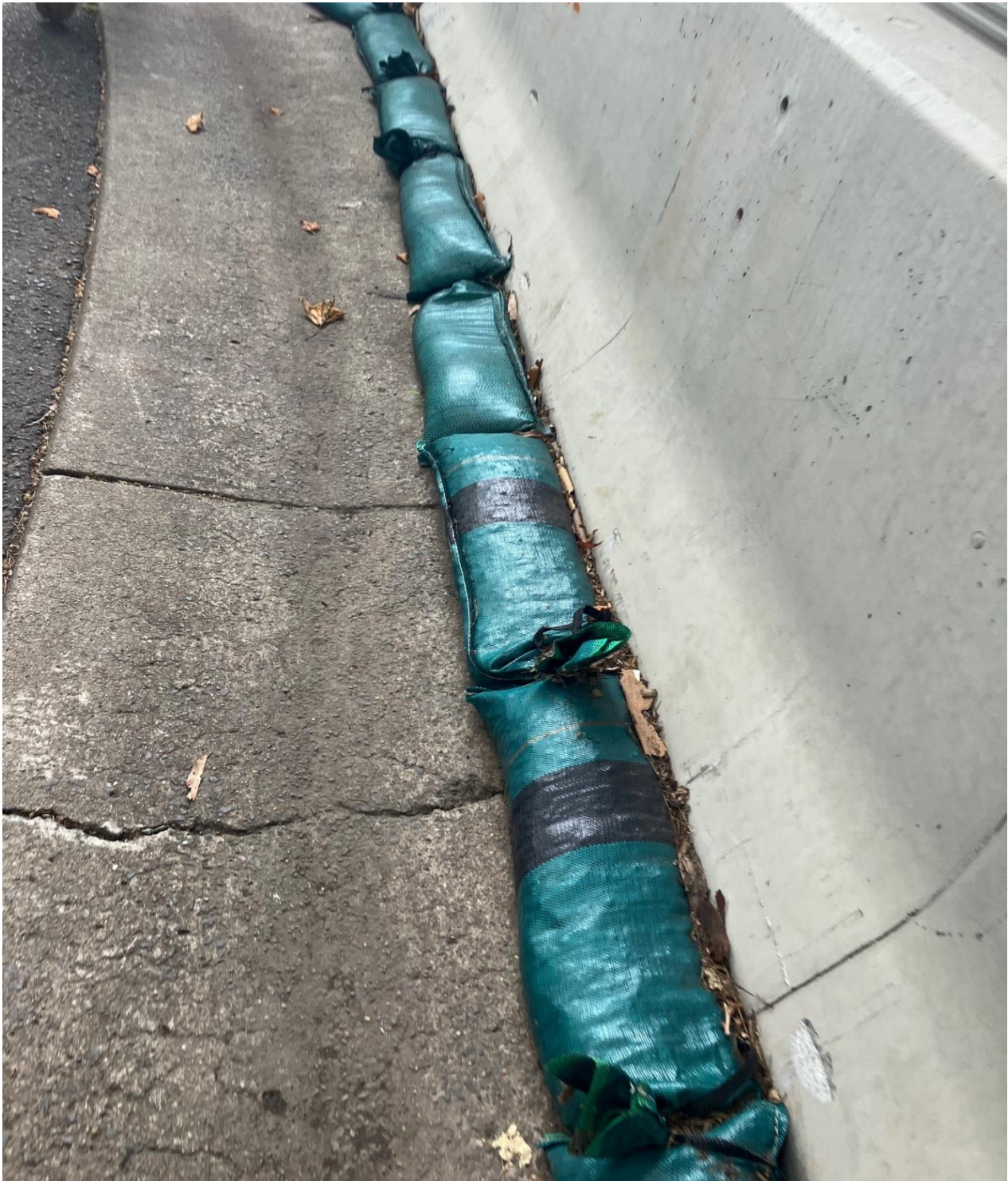
Sandbags installed at decline, Lambie Dew Drive
