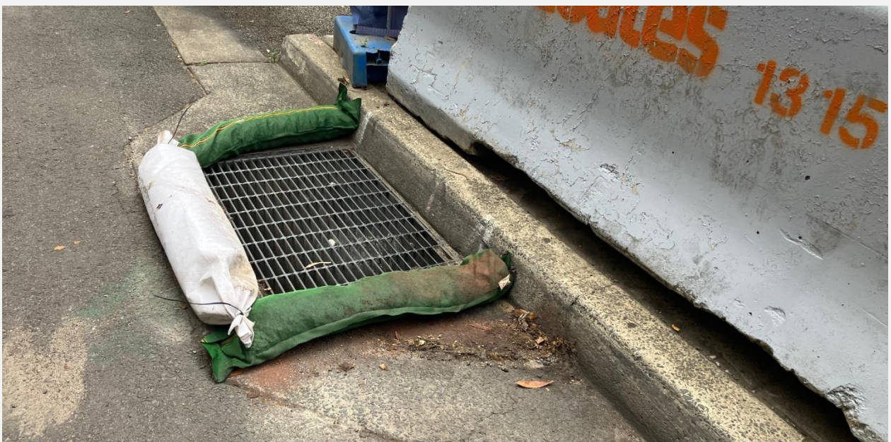
Protection of pit drains demonstrated at Lambie Dew Drive
