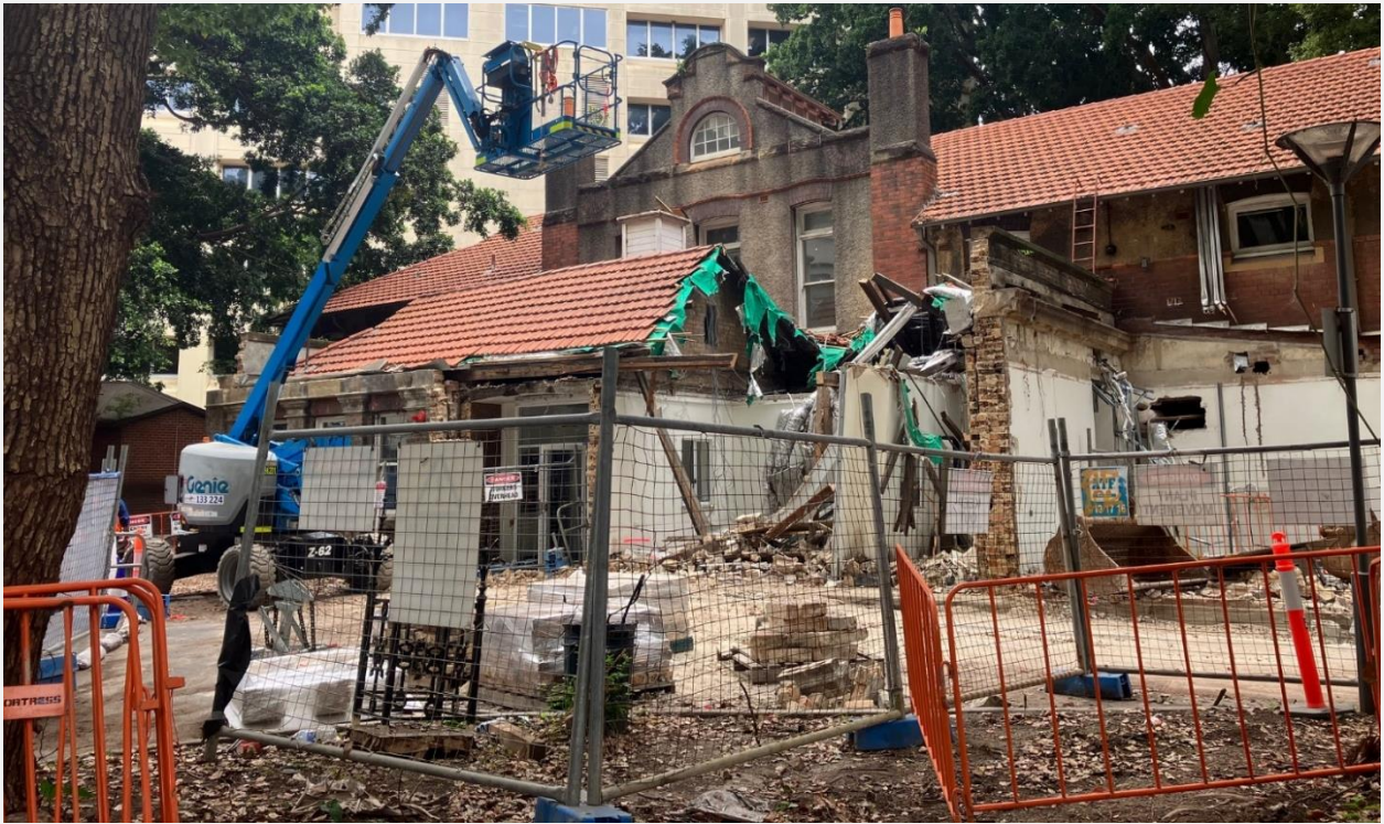
Demolition has commenced of Tissue Pathology and Diagnostic Oncology building.
