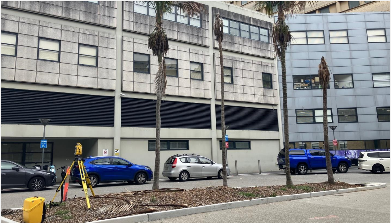
Current newborn & paediatric Emergency Transport Services entrance which will be temporary relocated under Stage 3.
