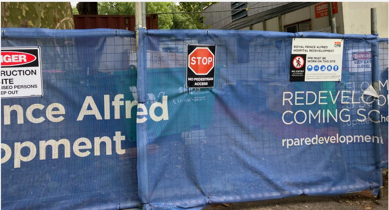
Demolition site at Lambie Dew Drive, fenced and secured.
