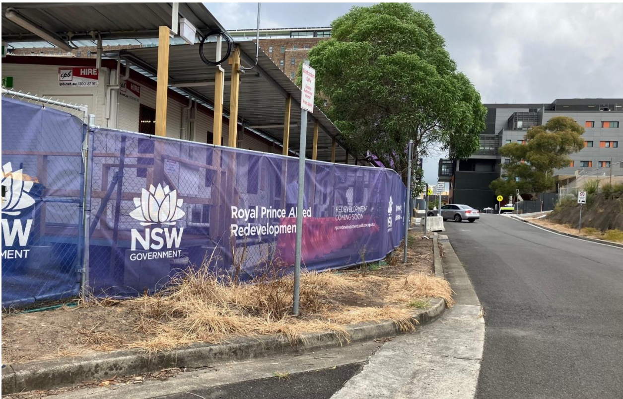
Shade cloth installed at main site compound, Hospital Road.
