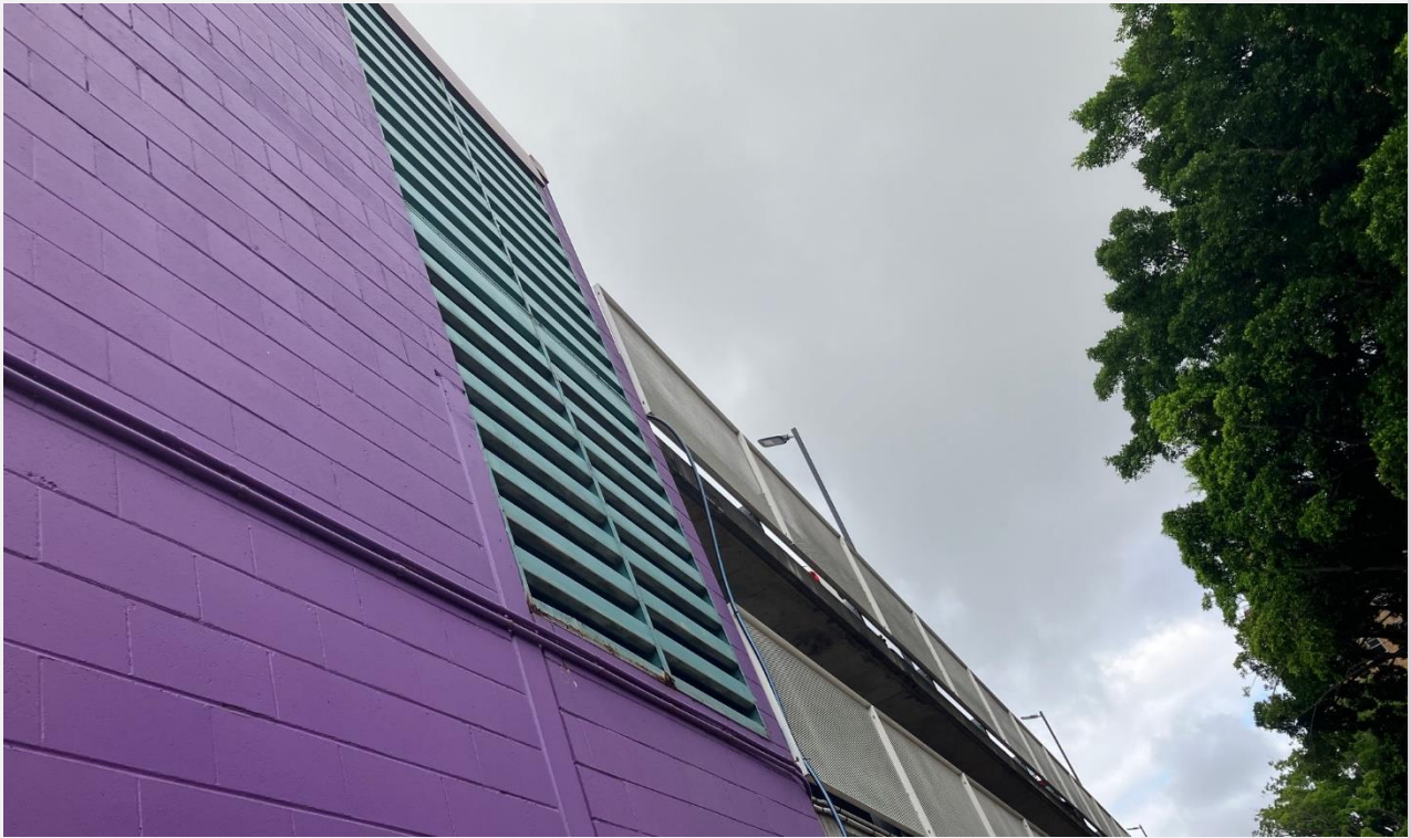
Car park where Temporary Helipad will be constructed.
