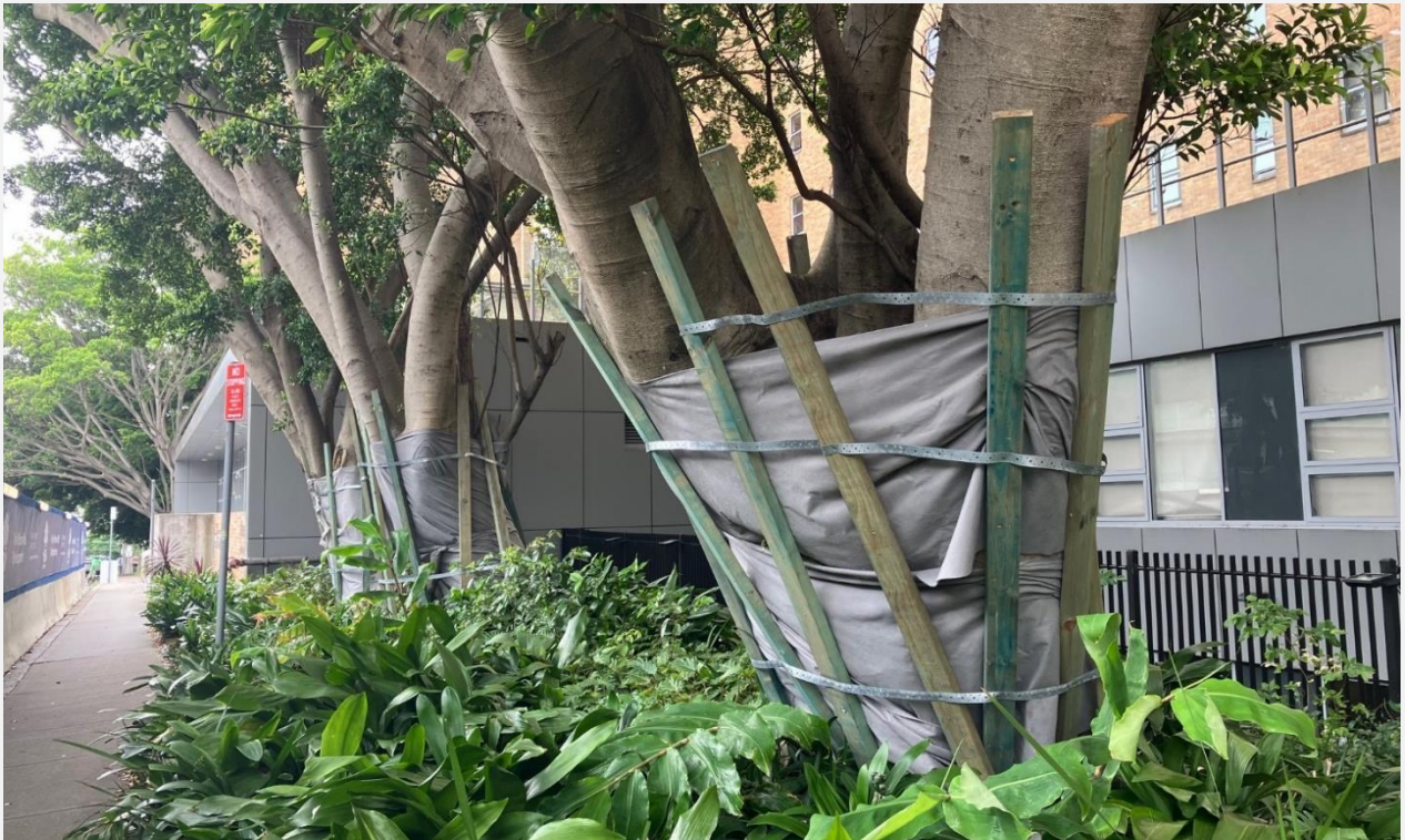
Tree protection installed adjacent to Temporary HLS. No other tree protection is required for the project.
