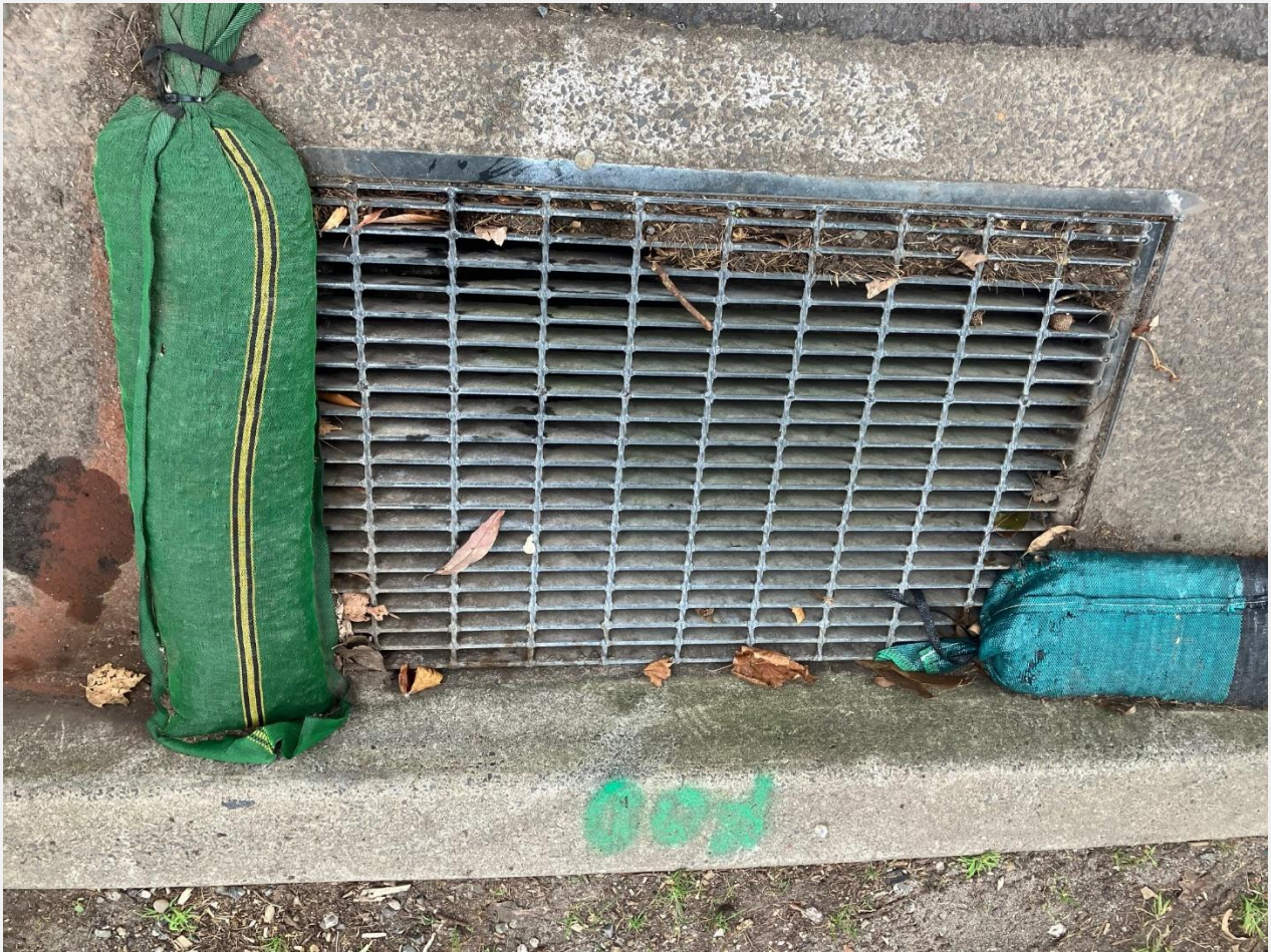
Protection of pit drains demonstrated at Lambie Dew Drive
