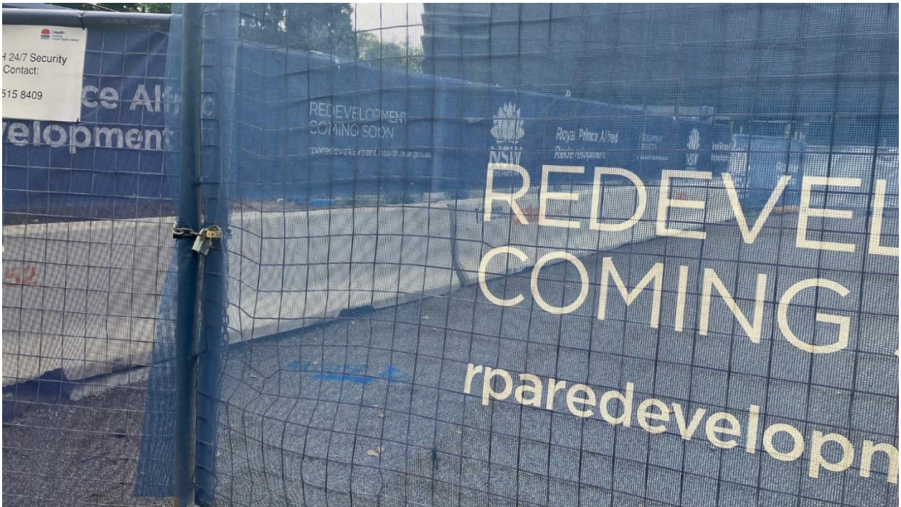
Locked gate for Ausgrid access as constructed by previous contractor
