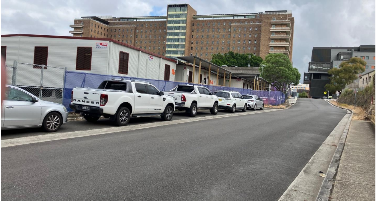
CPB main site compound located on Hospital Road. Road noted to be clean and clear of obstacles.
