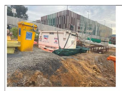
Improvements to refuelling pod and removal of impacted soil.
