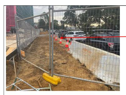
Exposed verge along Shoalhaven Street lacking erosion and sediment control (ESC), and vehicle impacting stormwater drain ESC.
