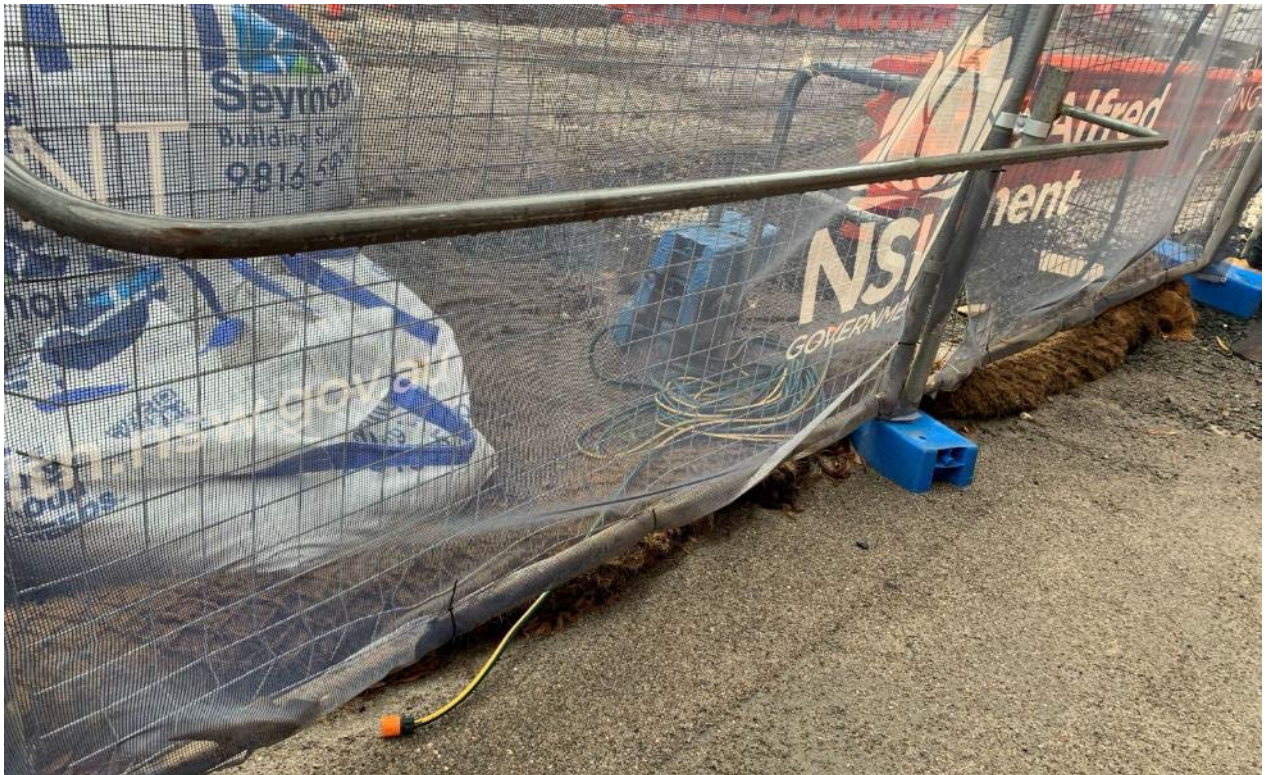
Coir logs in place at the boundary of the site.
