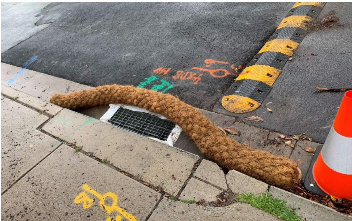
Controls in place for the stormwater drain pit.
