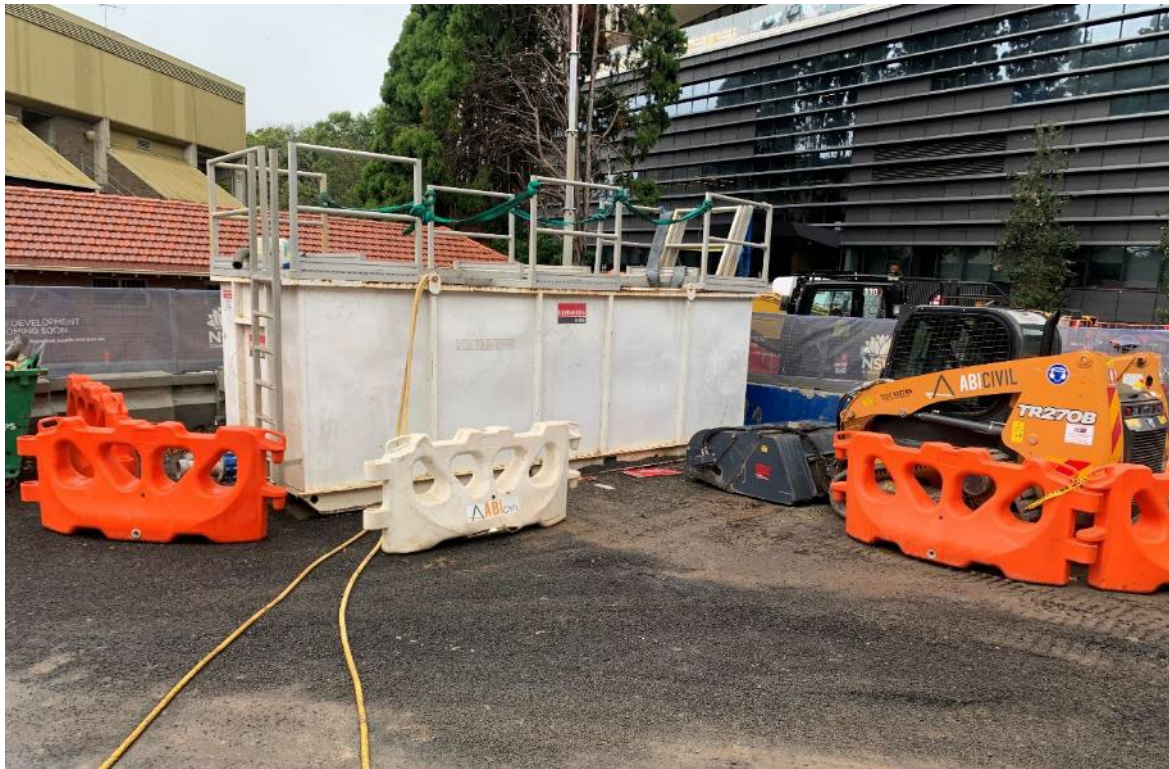
Rainwater collected in the site pumped out to the Sediment Tank before treatment.
