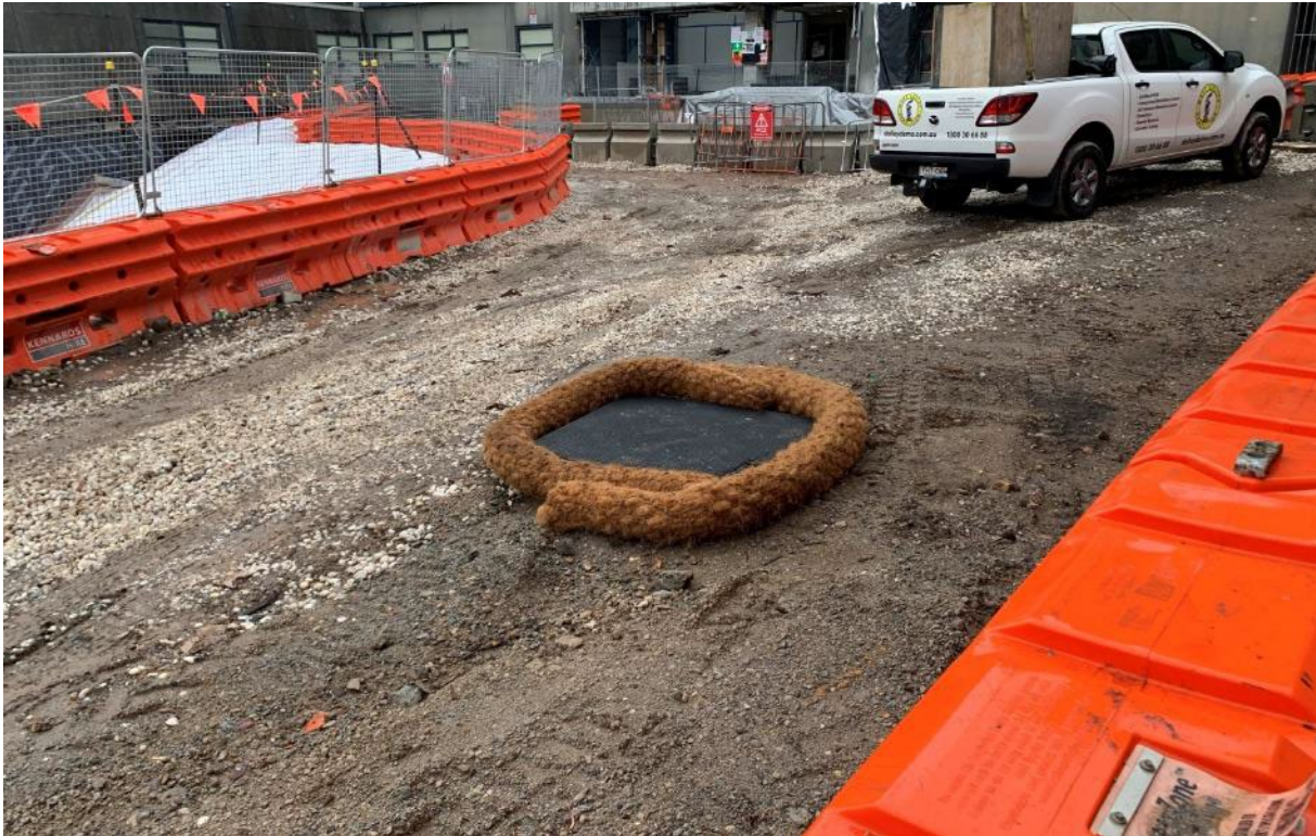
Controls in place for the pit drain.
