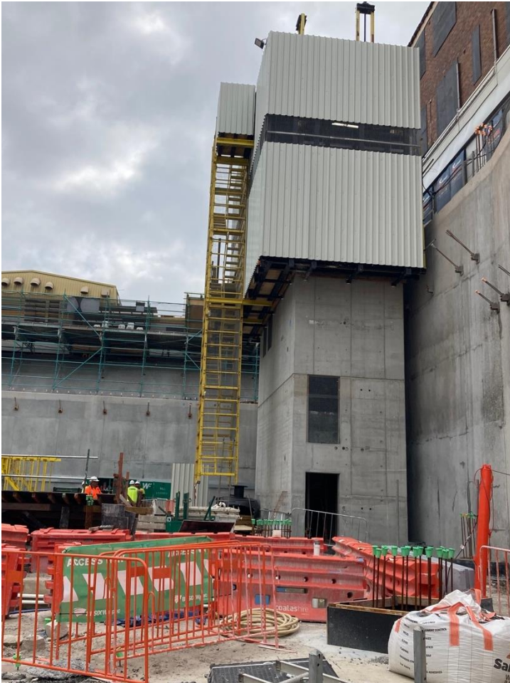
Photo 03 – Construction of building structure progressing – lift core.
