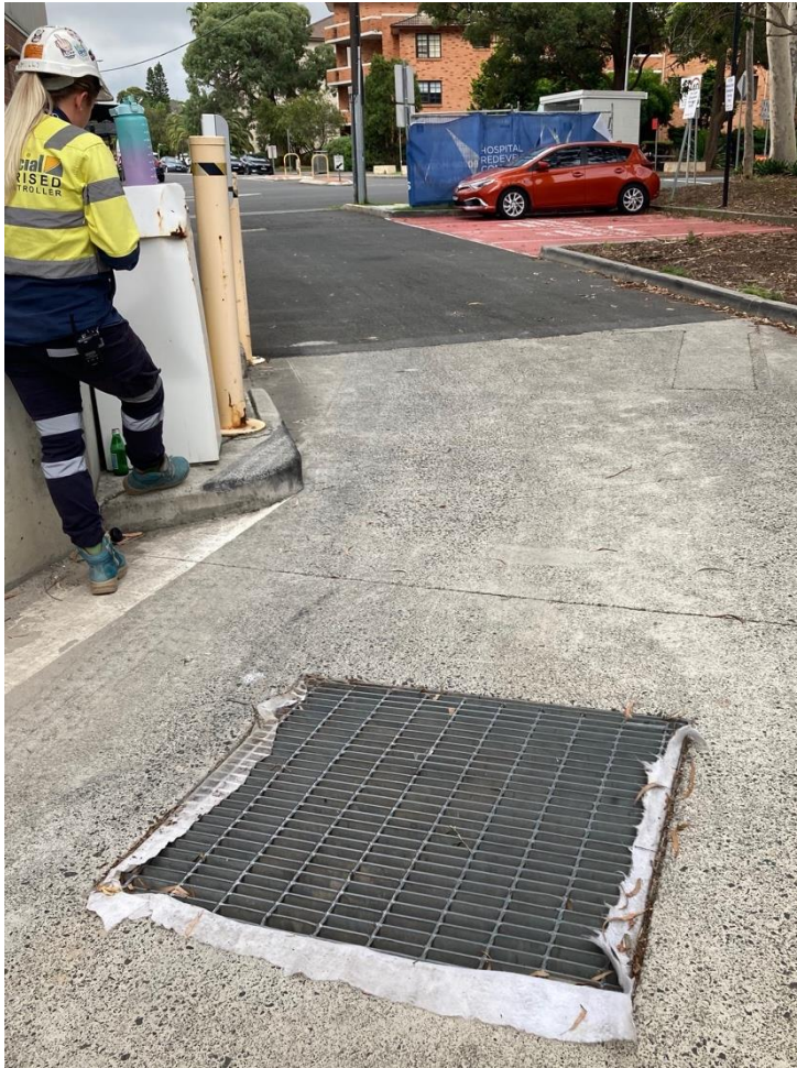
Photo 11 – Drains adjacent to construction areas covered with geofabric.
