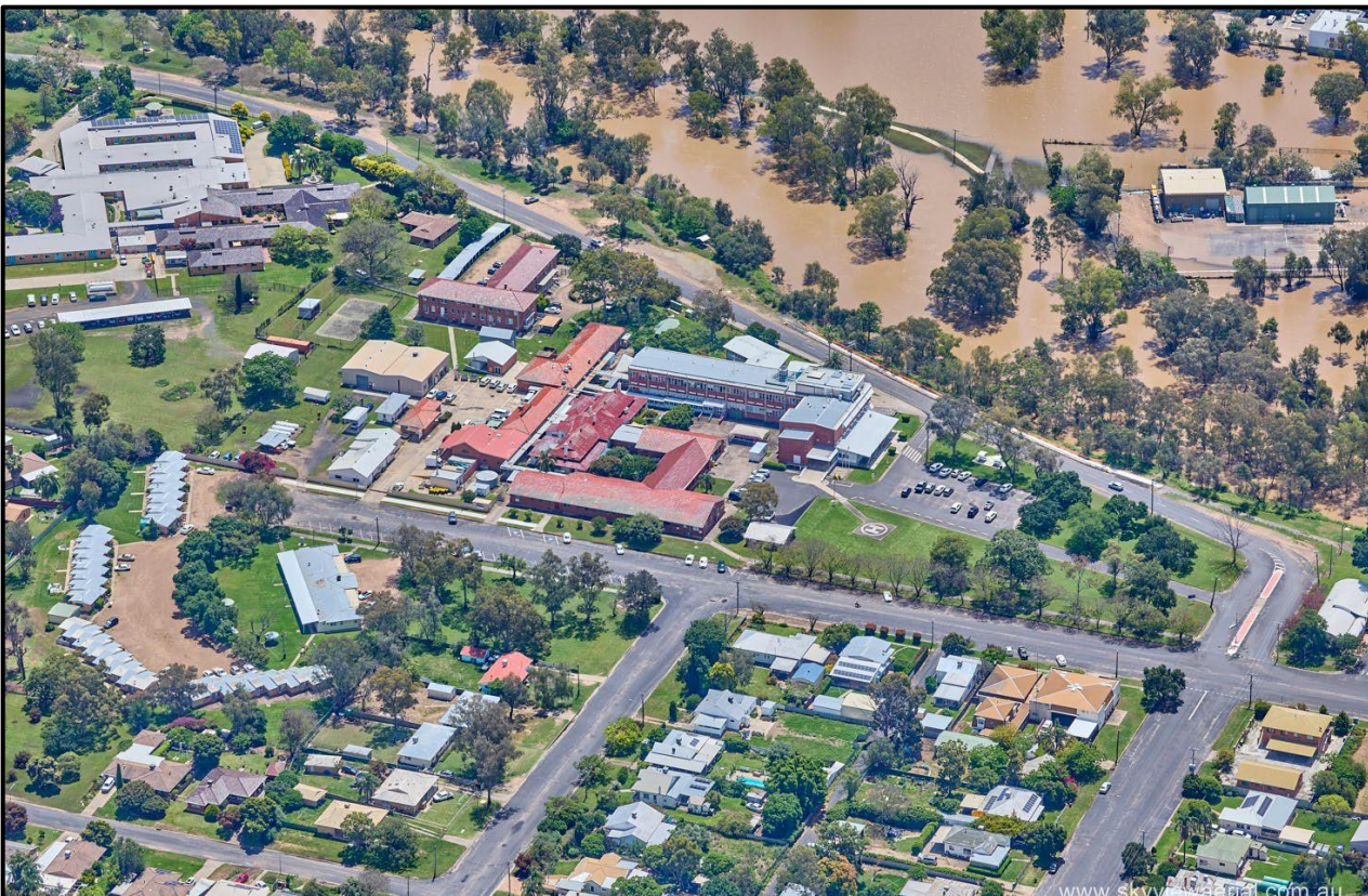
Figure 2 Aerial image of the site taken during a flood event in October 2022.
