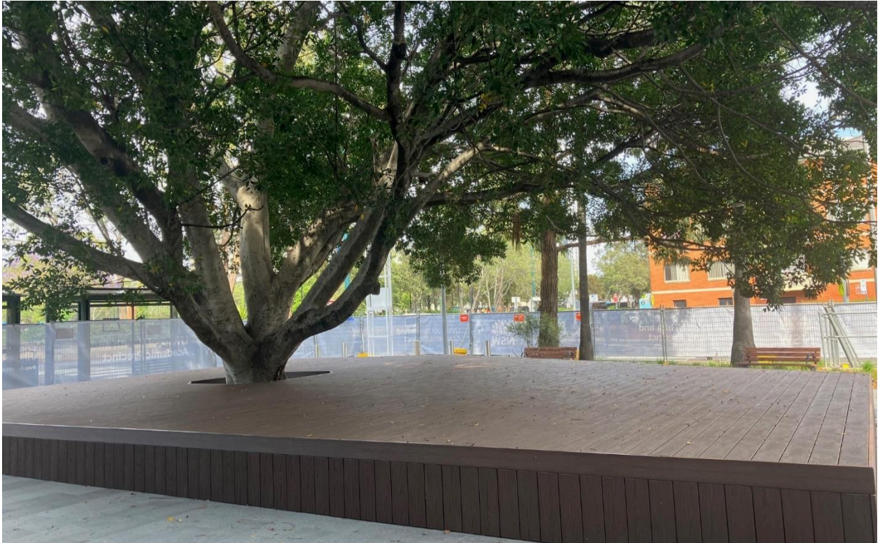
Retained tree with floating deck installed as per arborist advice.
