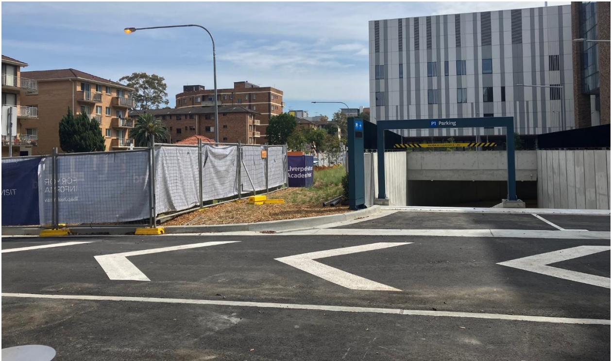
ISB parking. Some defects to address e.g., height of bar to be raised.
