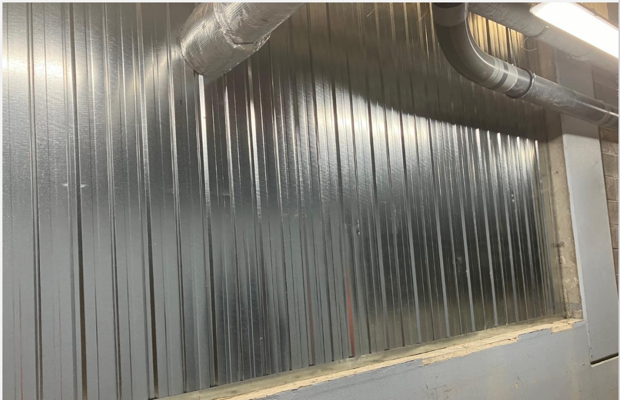
Fire wall installed at basement.
