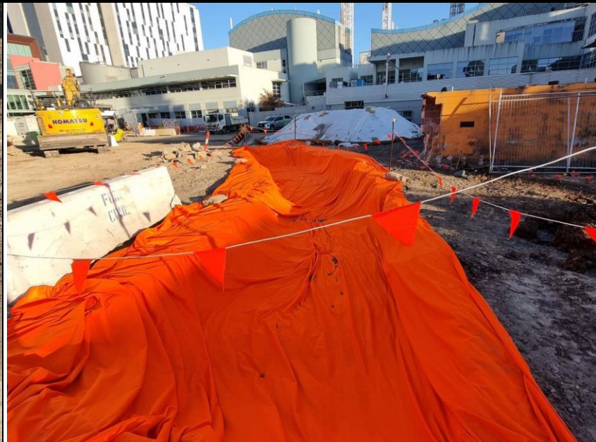
PHOTO 4 – INSTALLED GEOFABRIC MARKER LAYER IN FOOTING AREA
