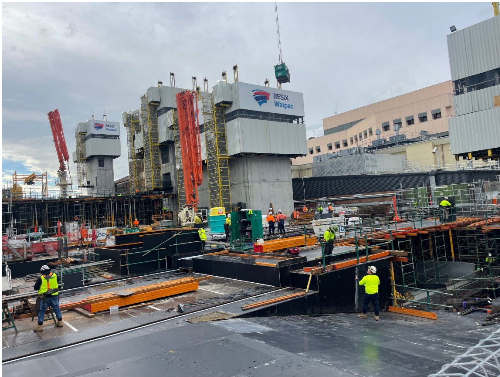
General site activities in progress. Note the progression of various jumpformwork.
