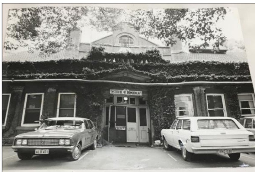
Figure 10. Photograph of the subject building, c.1970s (Source: "Survey of Hospital Buildings," The Royal Prince Alfred Hospital, May 1972, Royal Prince Alfred Hospital Archives)
