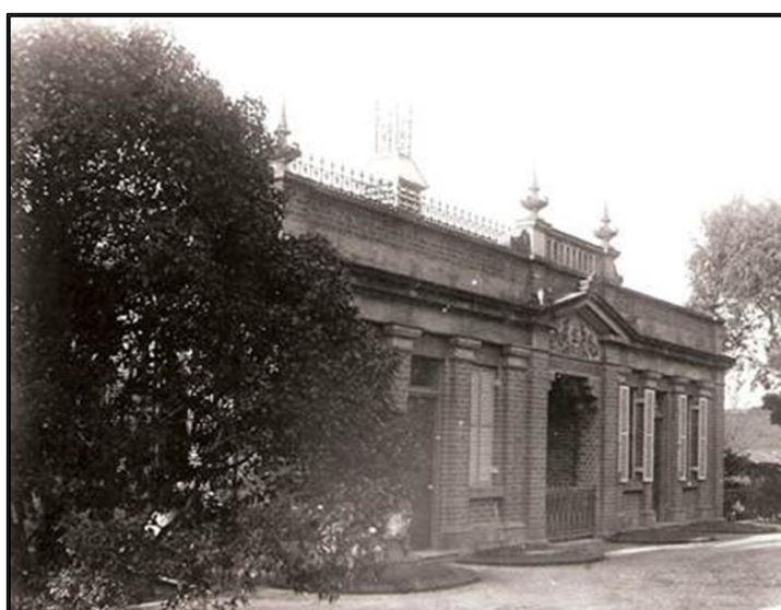
Figure 6. Early photograph (c.1903) of the primary façade. Note the external modifications include the removal of garden beds, doors and cresting (Source: RPA Archives)
