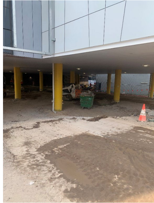
Site works, area watered down to reduce dust suppression
