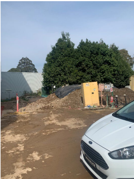
Materials stockpile, Dangerous Goods cabinet and fire extinguisher in place
