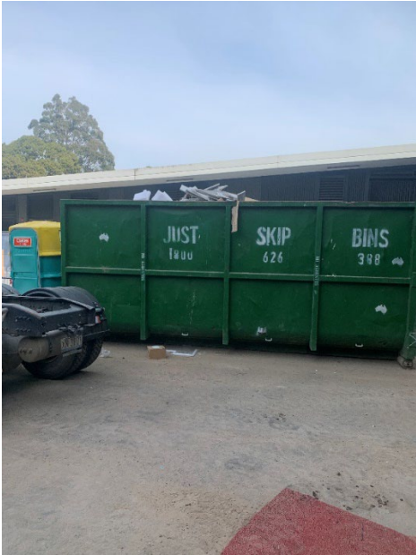
General waste skip bin being utilised to remove waste from site
