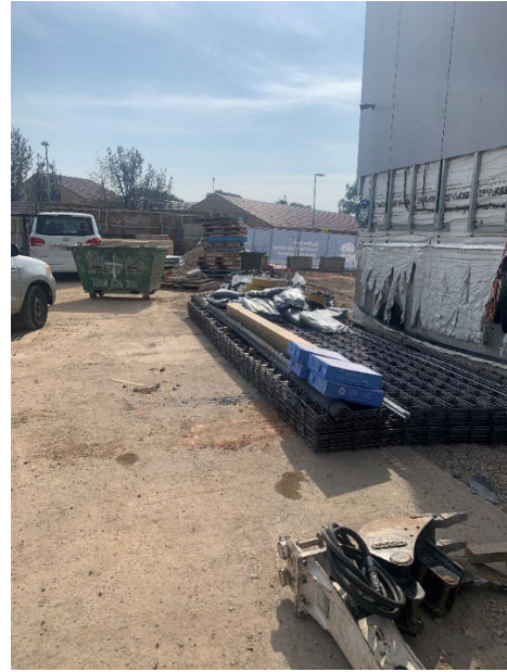
Site works (laydown area with general waste skip bin available)
