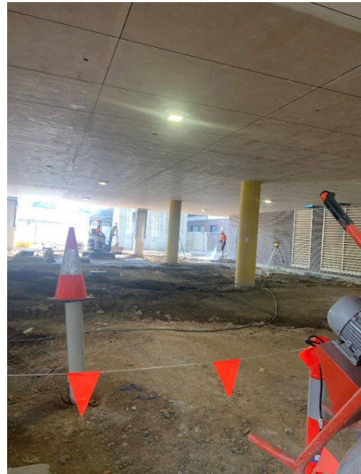
Minor earthworks, dust suppression with handheld hose
