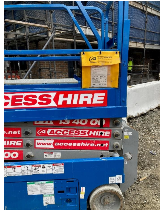
Photo 10 – Plant and equipment onsite registered and maintained.
