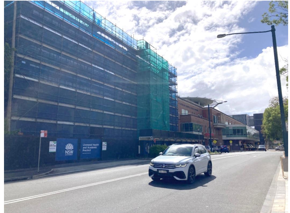
Photo 2 – Hoarding and scaffold adjacent to hospital on Elizabeth Street
