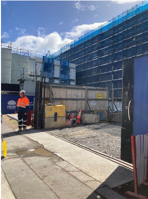
Photo 5 – Traffic controllers present to manage construction vehicles access.
