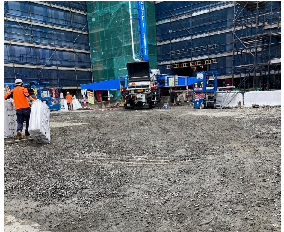
Photo 4 – Vehicles contained within the site. Rumble grid at vehicle access point.
