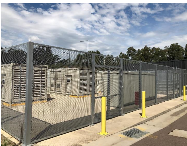
Diesel backup generators and diesel supply in locked bunded area
