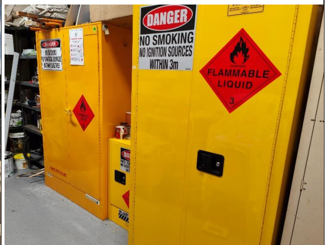
Locked and bunded chemical storage area
