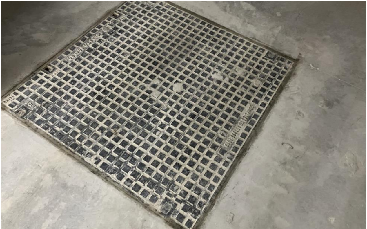
Water is collected onsite into a tank (located here) which is tested prior to discharging.
