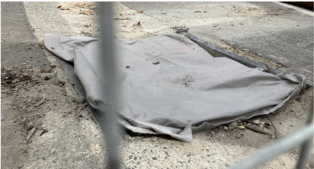
Pit drain covered in geofabric
