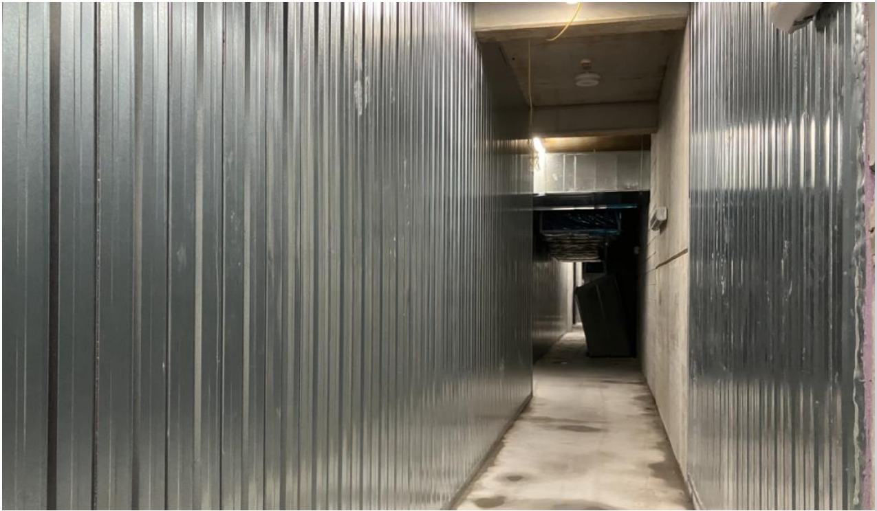
Fire safety wall installed at basement
