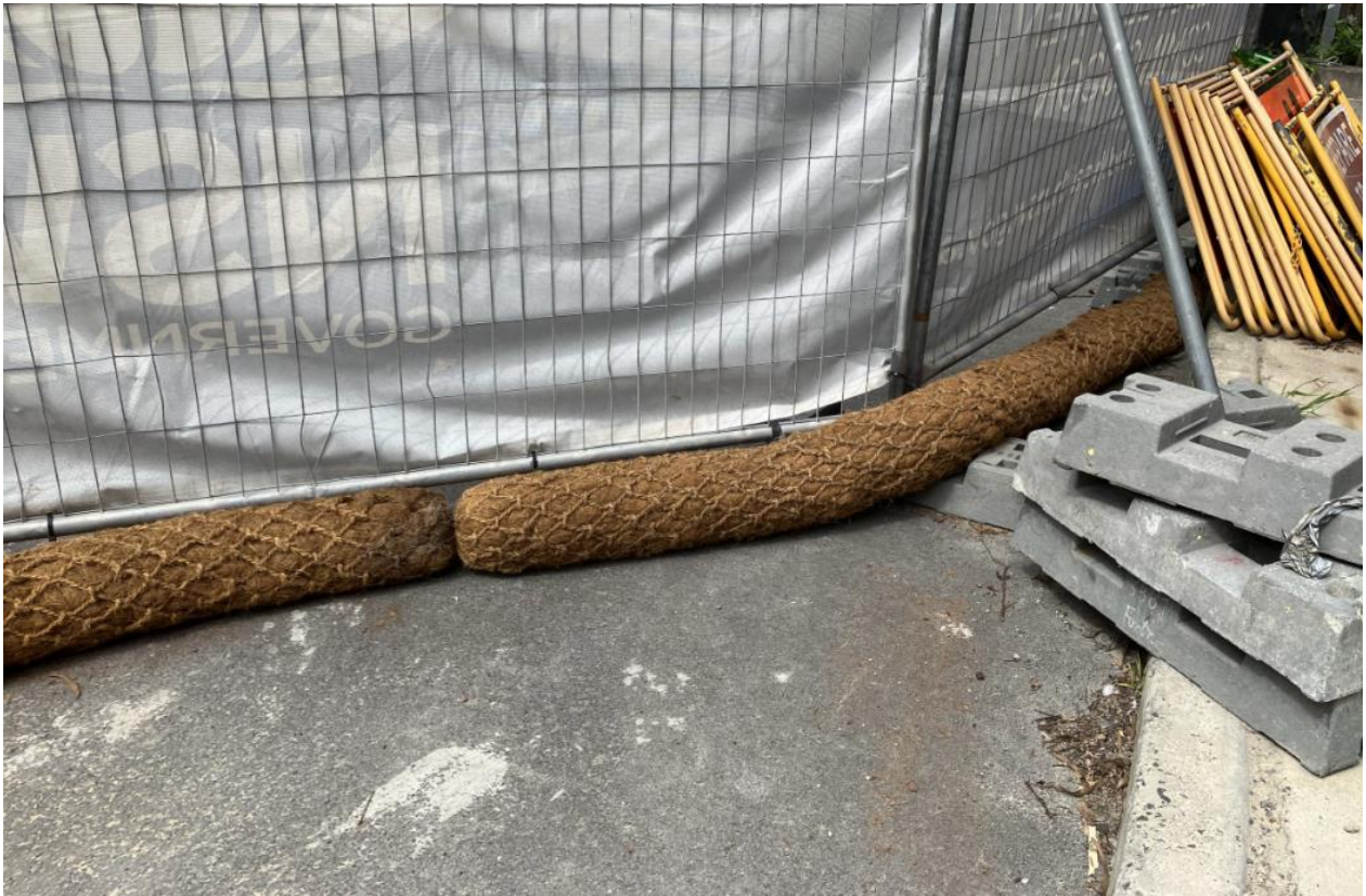
Coir logs in place at lowest point of site which leads to stormwater drain (below)
