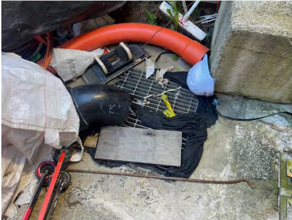
Image 9: Onsite stormwater pit requiring cleaning and reinstatement of controls.
