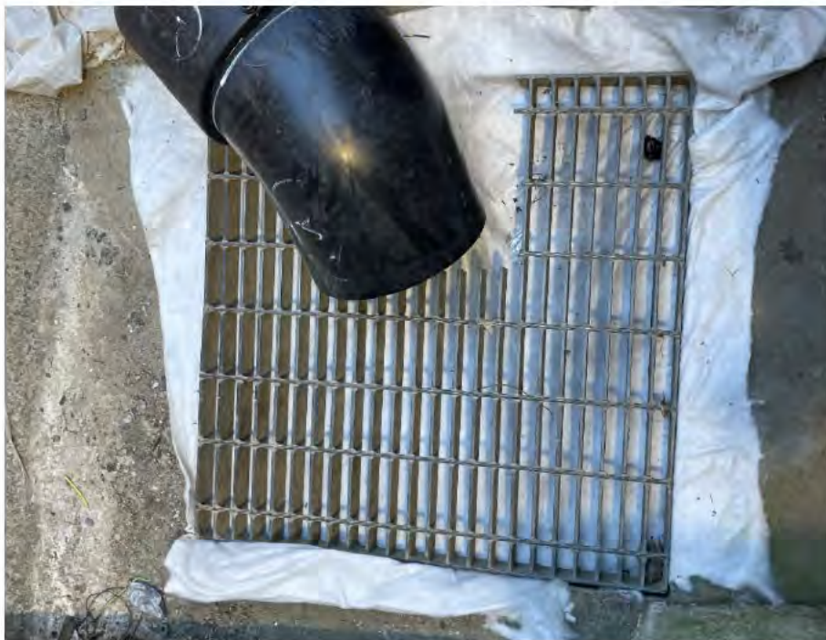
Image 9: Onsite stormwater pit requiring cleaning and reinstatement of controls.
