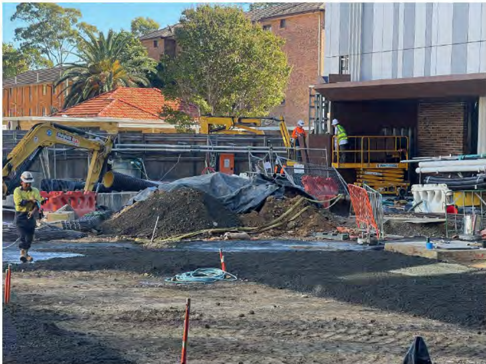
Image 8: Topsoil being temporarily stockpiled and covered in plastic.
