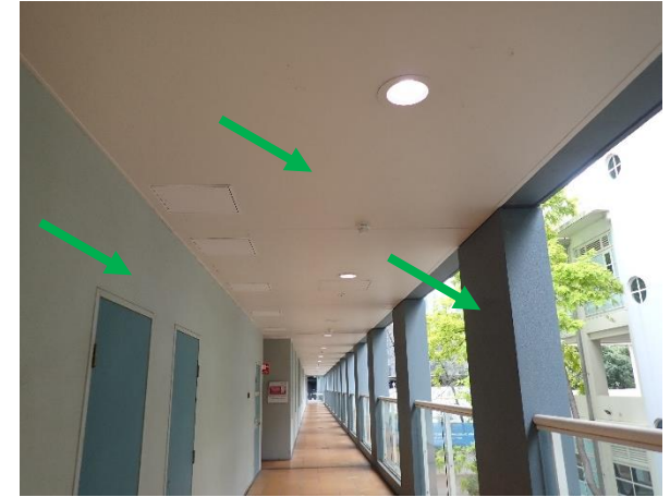
Photo 21: Level 2 Linkway and Pathway, external area, ceiling– non-asbestos fibre cement. Non-lead based light blue paint on cement rendered walls and non-lead based dark blue paint on pillars
