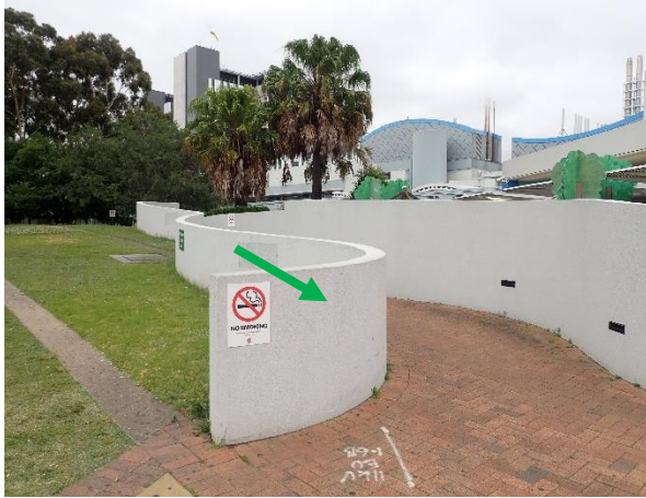
Photo 31: Level 2 external forecourt, curved walkway walls– non-lead based grey paint
