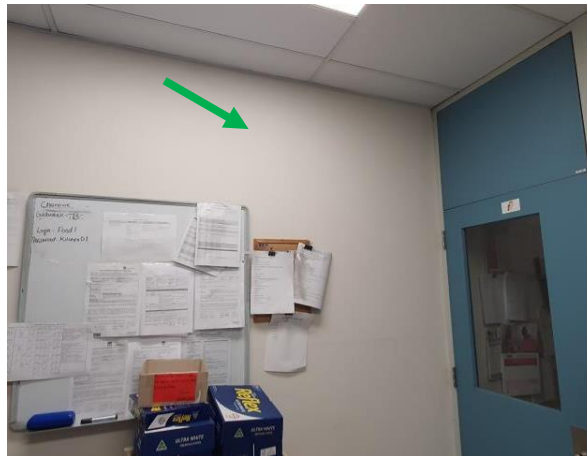
Photo 11: Level 1 Kitchen, cement rendered walls – non-lead based white paint
