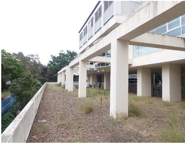
Photo 25: Overview of Level 2 Pathology expansion area
