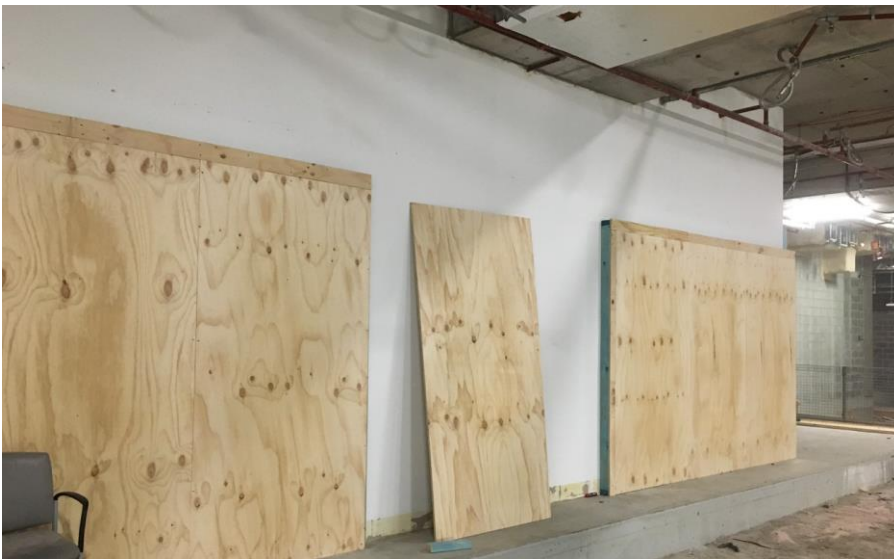
Figure 3: Temporary acoustic barrier - VVMF site
