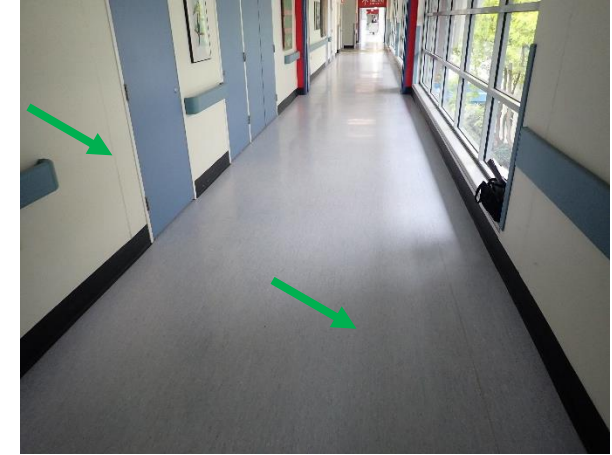
Photo 33: Level 3 Linkway and pathway, internal area throughout, flooring – assumed non-asbestos blue vinyl flooring. Walls and door jambs – non-lead based white paint
