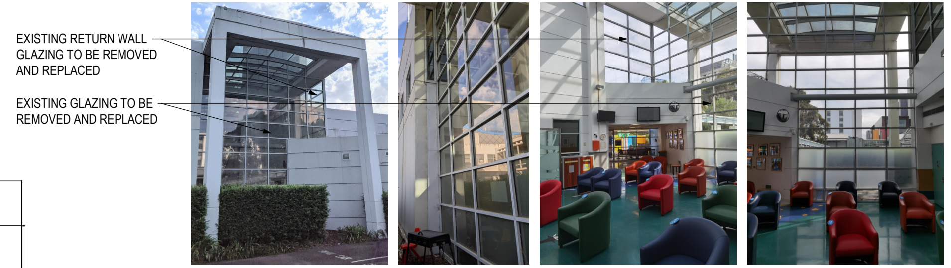
EXISTING CONDITION VIEWS
