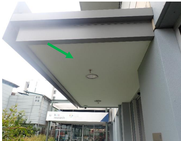
Photo 29: Level 2 Clinical Research Centre (CRC), soffit lining – non-asbestos fibre cement
