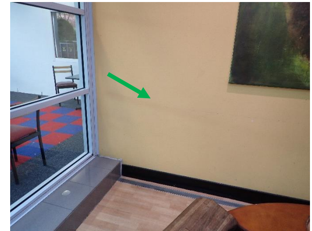
Photo 6: Level 1 Galleria entrance, cement rendered walls – non-lead based yellow paint
