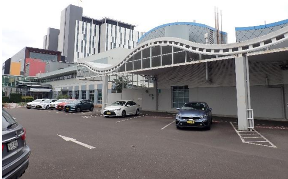
Photo 28: Overview of Level 2 External Forecourt
