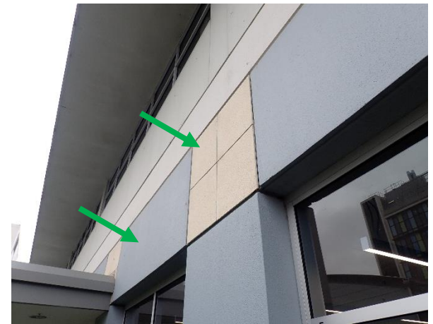
Photo 30: Level 2, Clinical Research Centre (CRC) façade– non-asbestos compressed fibre cement. Walls, non-lead based blue paint
